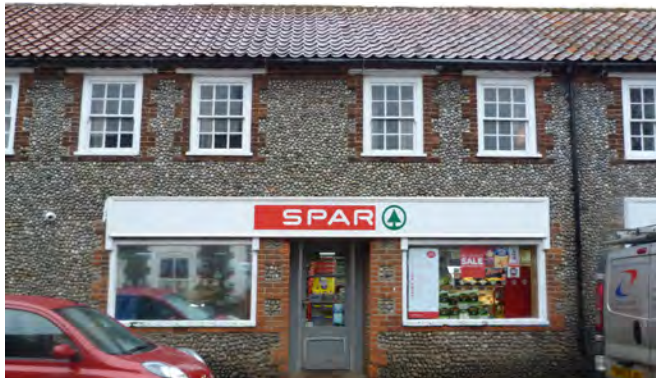
Spar, located in a former cottage along Westgate Street
