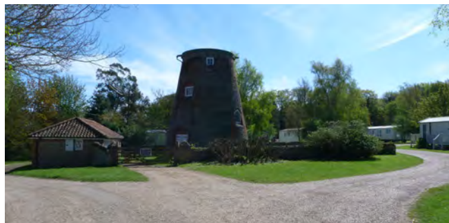
The former mill within the caravan site
