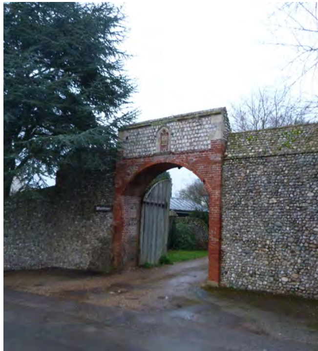
Gateway to Whitefriars and wall at the north end of Back Lane, with sloped flint capping detail
