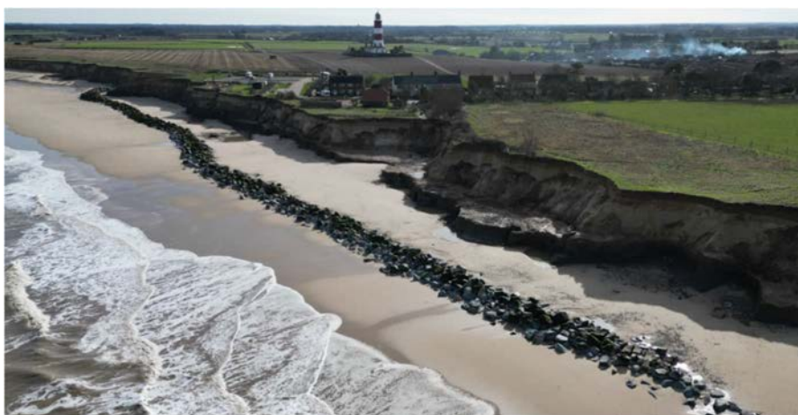
Figure 5-6. Happisburgh rock bund (North Norfolk District Council, Drone Footage from 27th Feb 2024)
