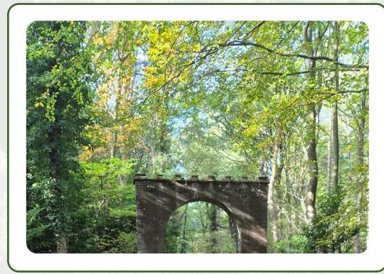
The arch was restored and the crenulated capping stones replaced with copies. The original stones were Gritstone and replacements are precast concrete. To the south of the arch is an old fish pond which now makes up the amphitheatre. Interpretation for the arch, explaining its existence, is on the work plan to be completed.
