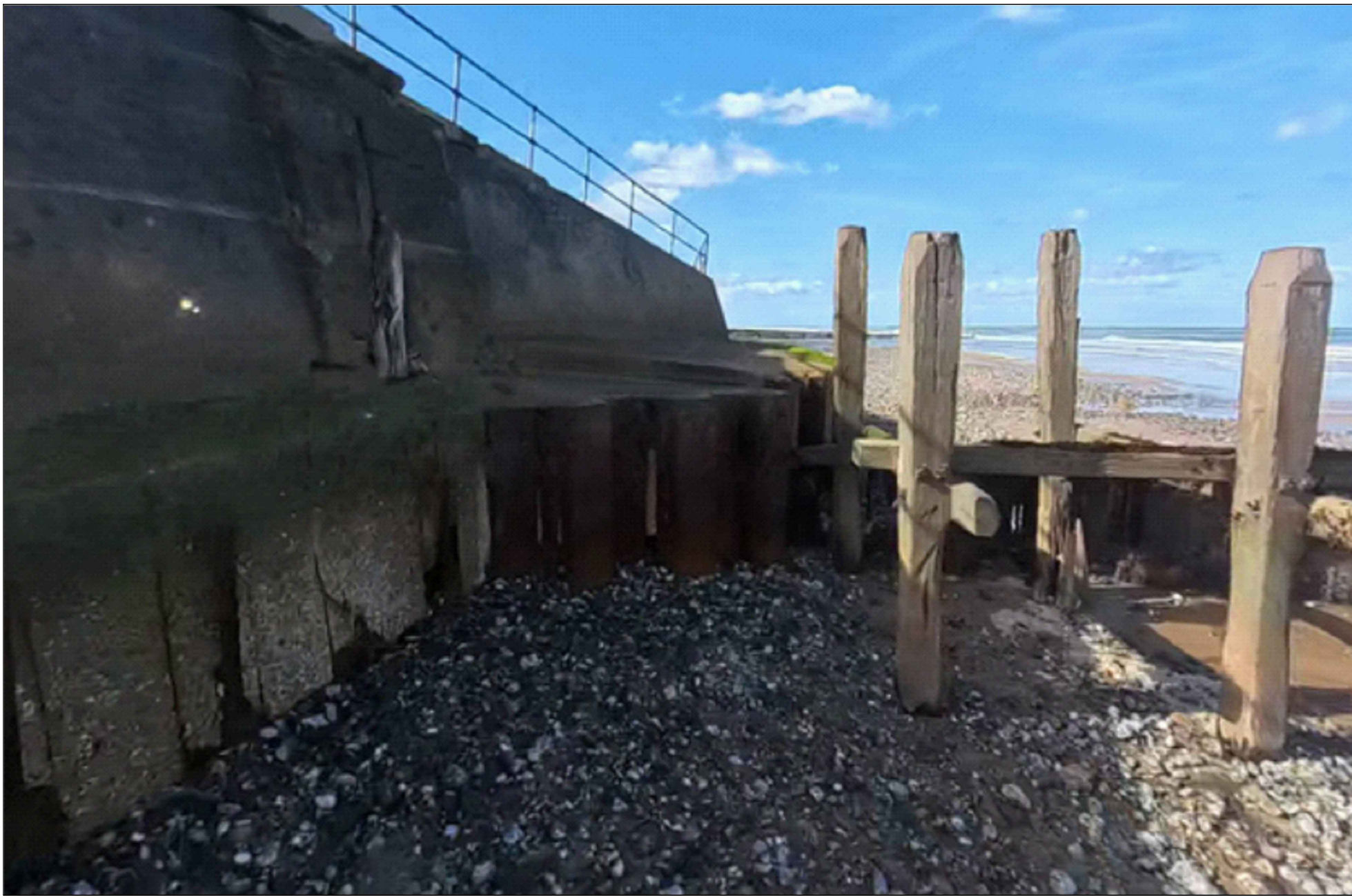
PHOTO 3 - TIMBER PILE REMOVAL
