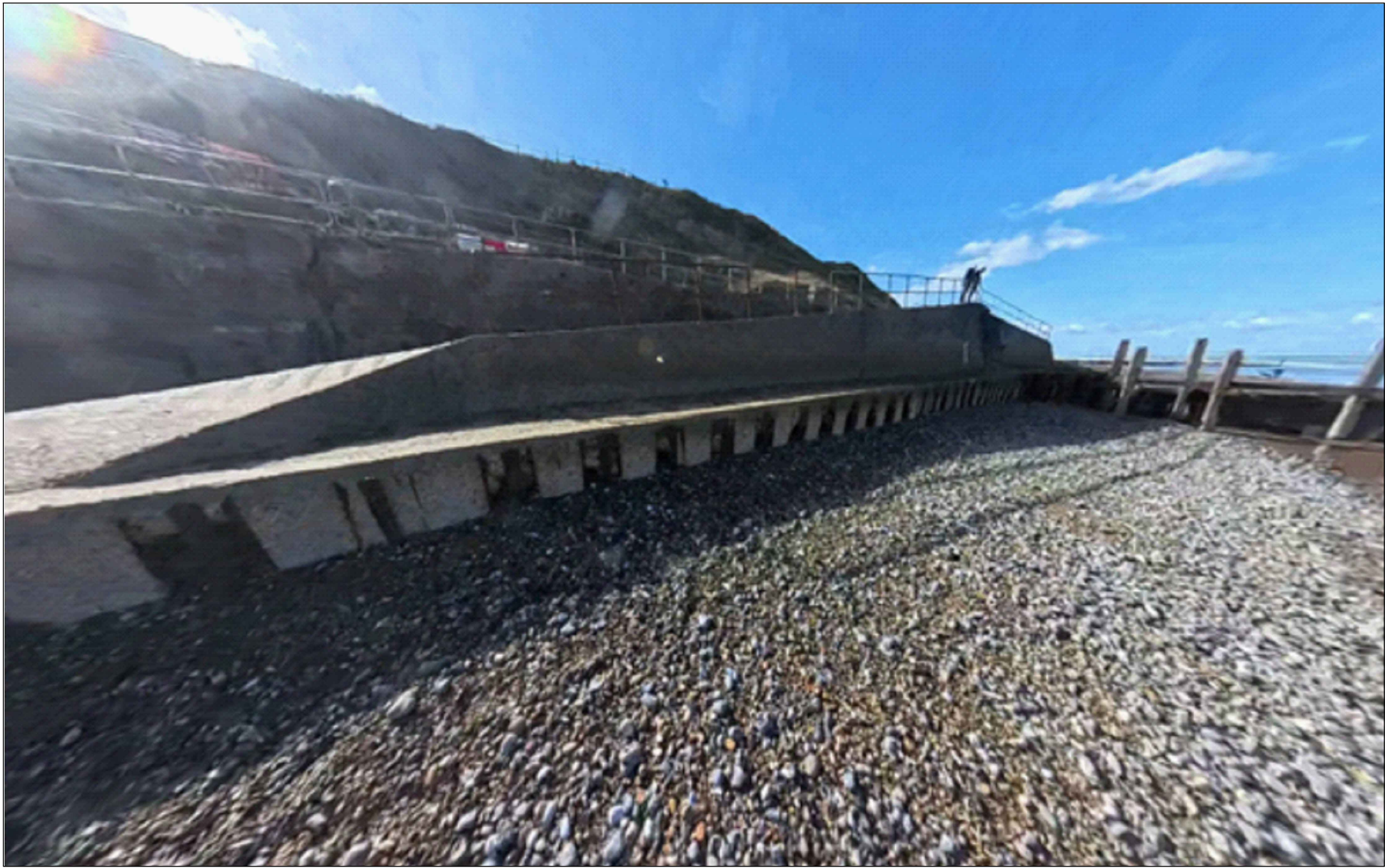
PHOTO 4 - EXISTING PILE LINE
