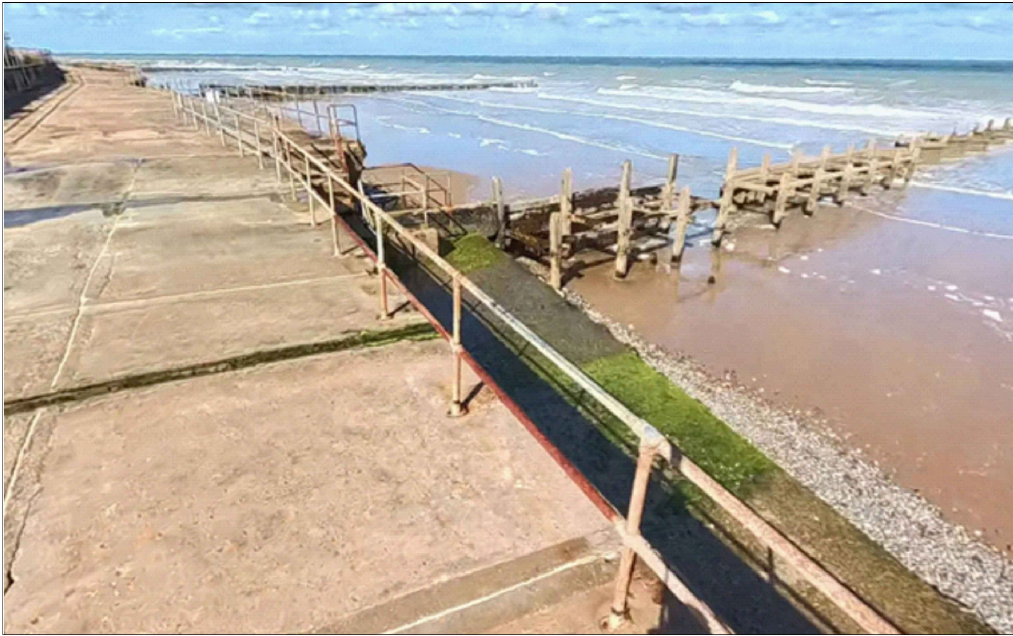
PHOTO 6 - TIMBER PILE REMOVAL
