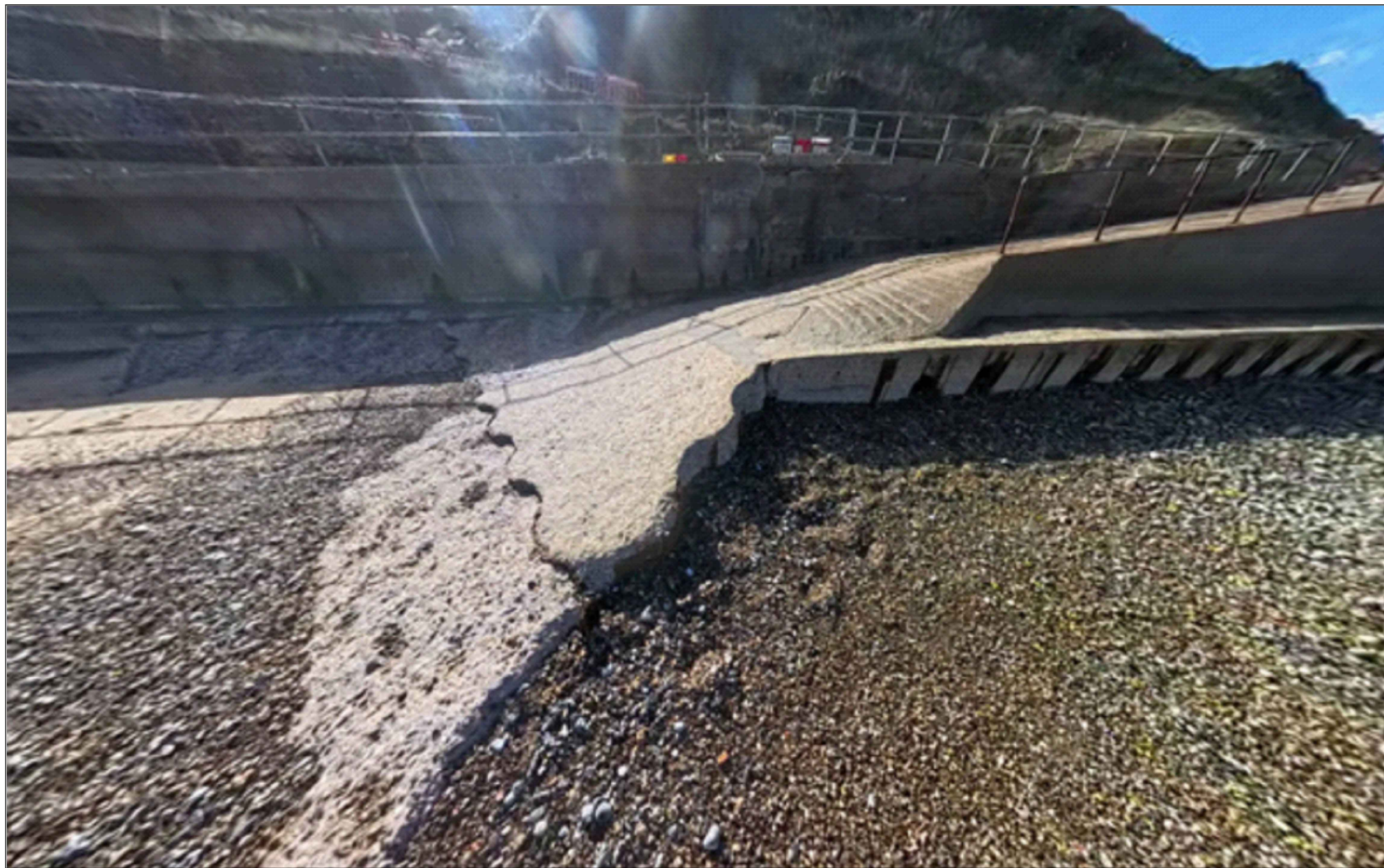
PHOTO 2 - WEST TIE IN LOCATION
