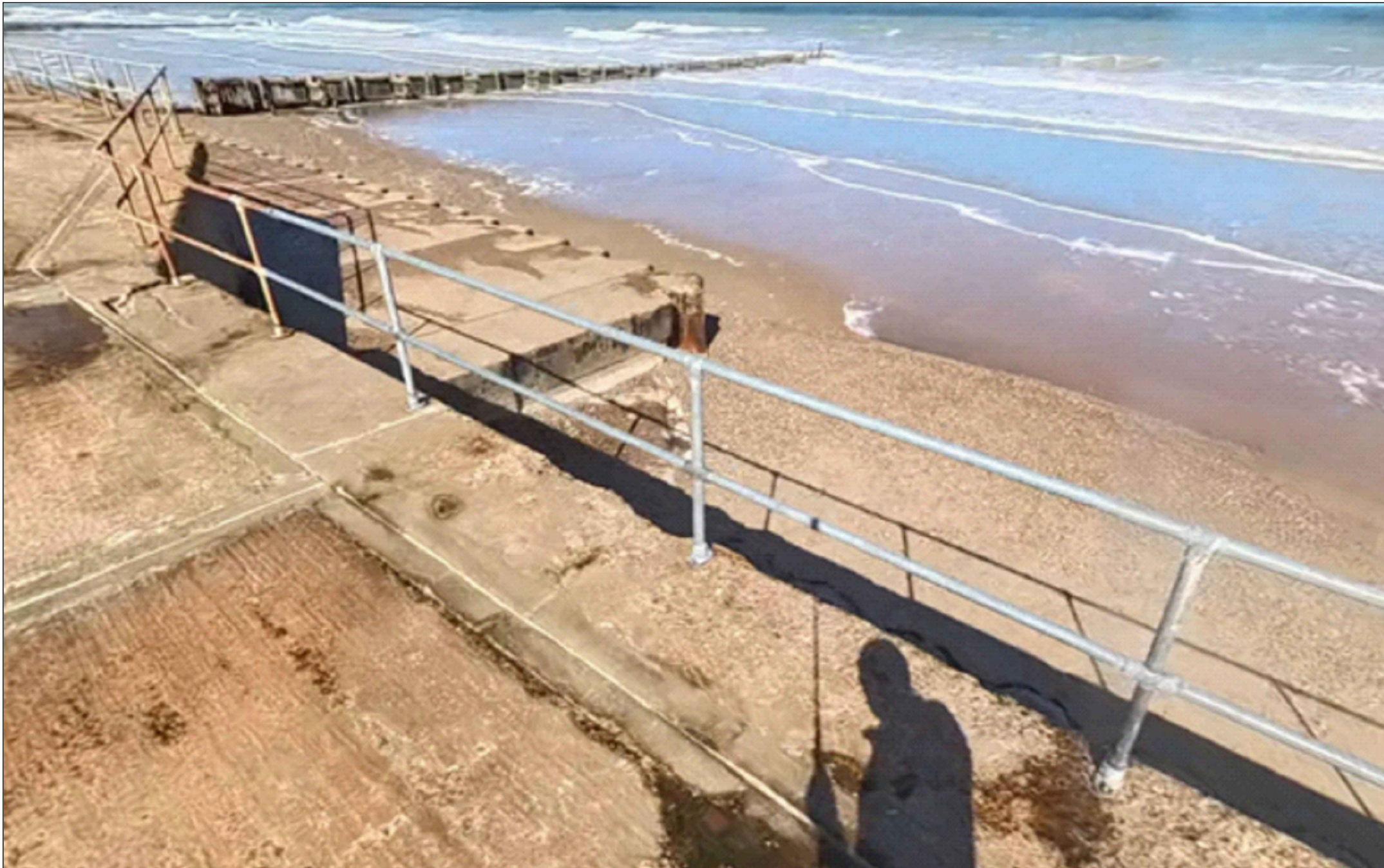
PHOTO 5 - WEST TIE IN LOCATION
