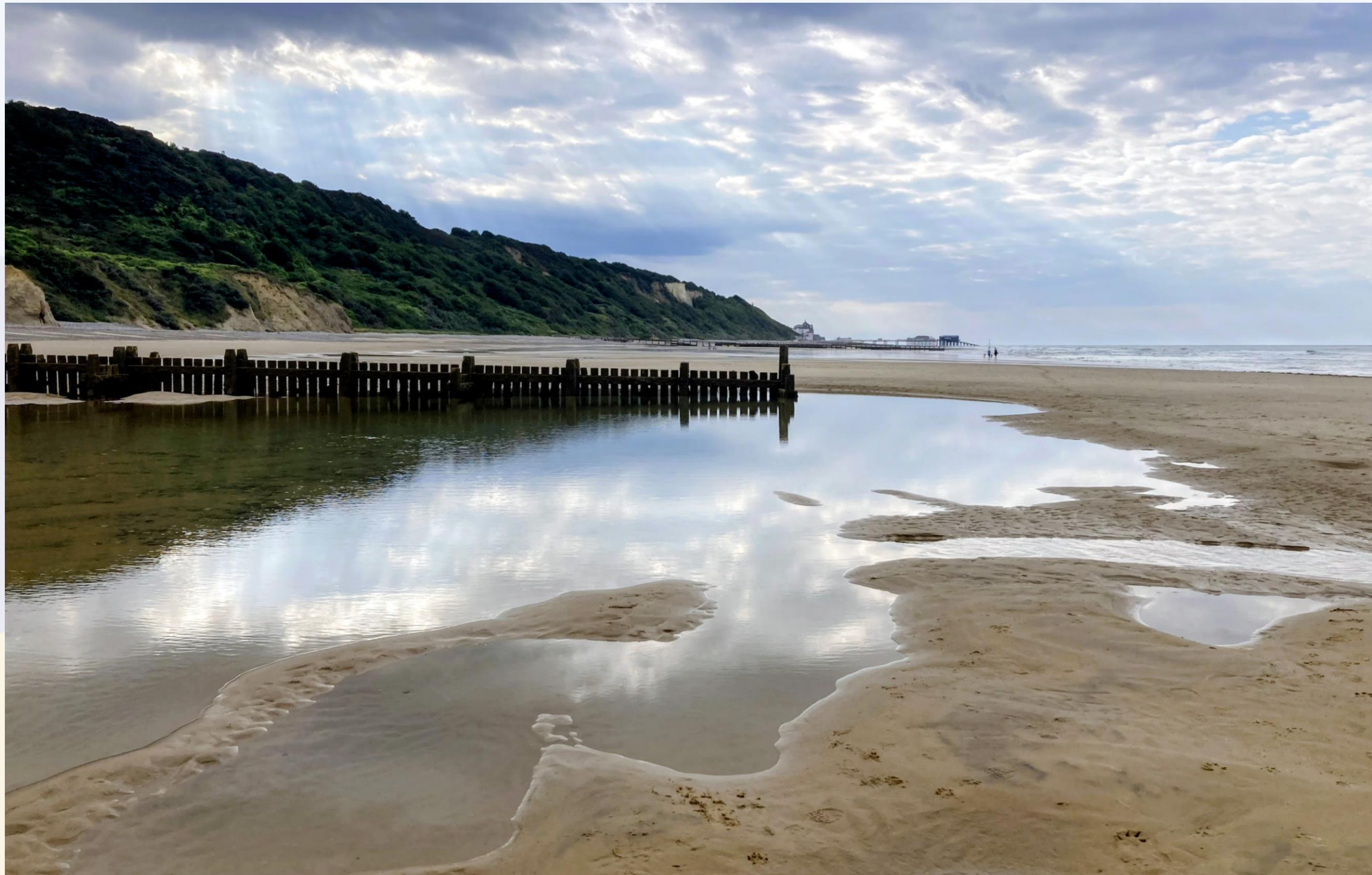
Figure 32: Overstrand beach featuring timber Groynes. Image taken by JBA Consulting, September 2025.
