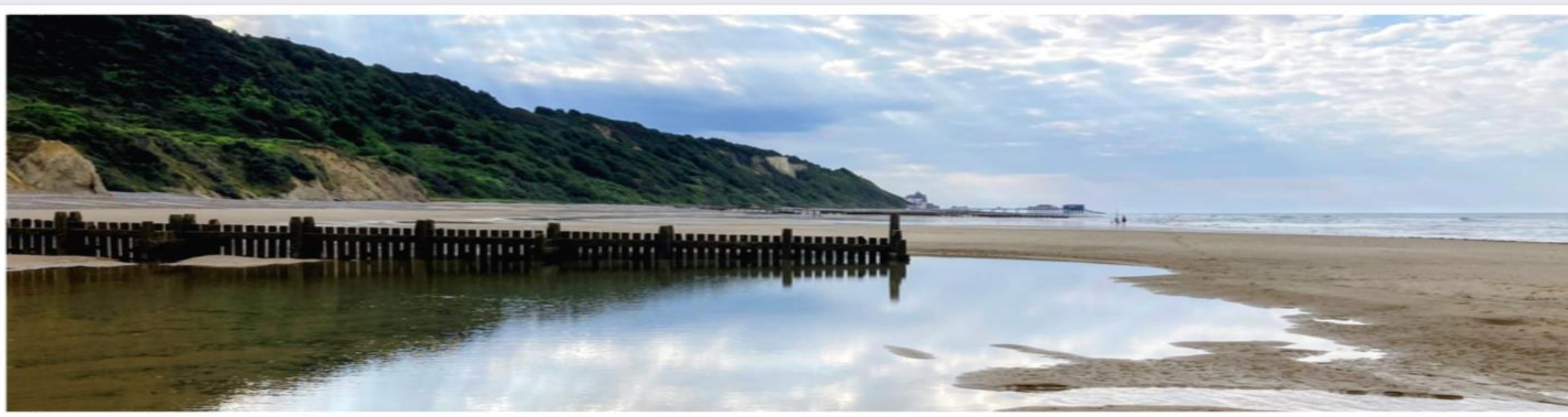
Figure 27: Overstrand beach featuring timber Groyne. Image taken by JBA Consulting, September 2025.
