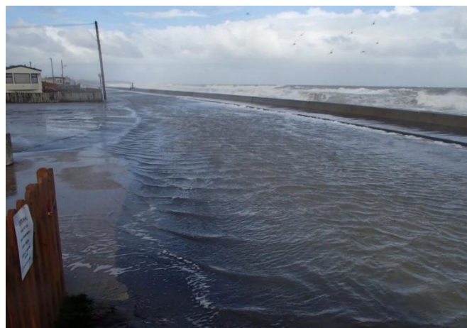
Flooding at Walcott during the 2013 storm surge (North Norfolk District Council)
