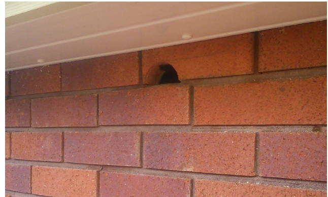
Figure 29: Example of a Swift brick under an eave.
