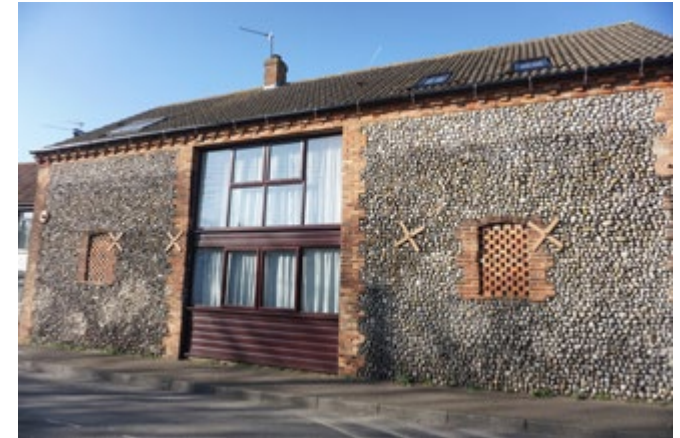
Converted barn on Valley Lane
