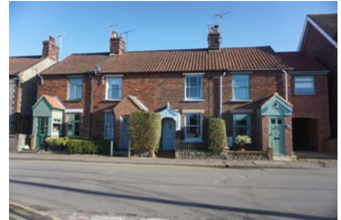
Victorian cottages on New Street
