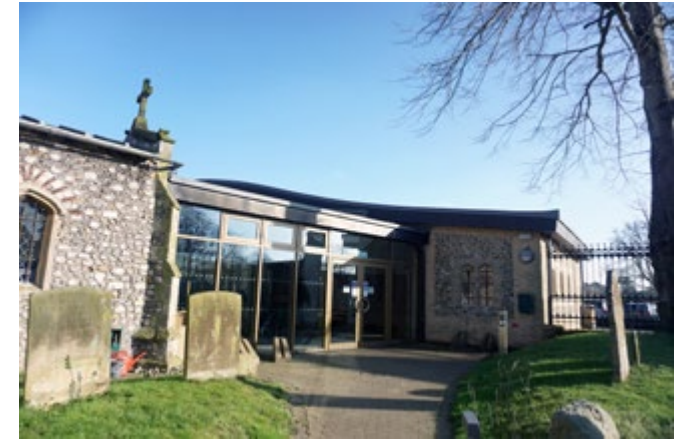
Extension to St. Andrew's Church
