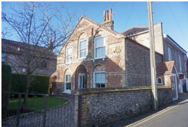
Converted Corn Hall on Albert Street
