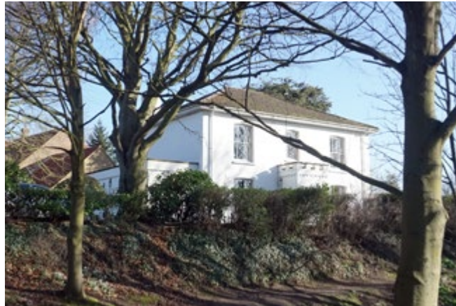
Early-twentieth century house adjacent to the Horn Pits newly included within the Conservation Area boundary (area G on the plan)
