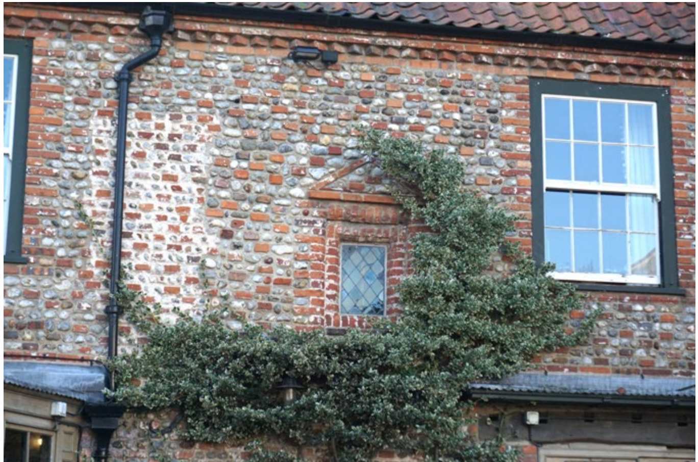
Flint and brick chequer pattern and small sixteenth century window on Byfords, Shirehall Plain
