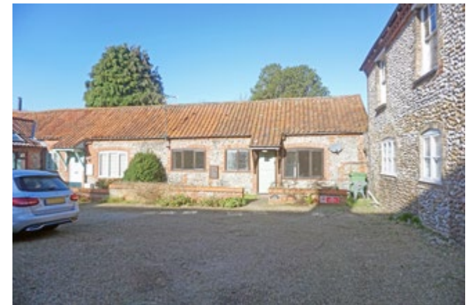
Converted outbuildings/stables off New Street
