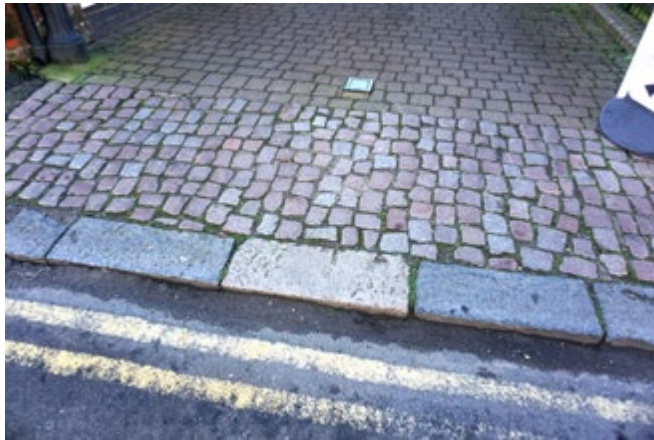
Granite kerb stones, granite setts and brick pavers on New Road, with double yellow lines
