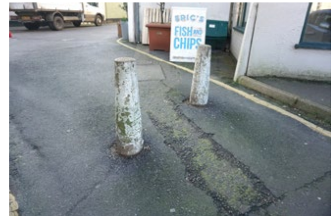
Unattractive concrete bollards on Fish Hill
