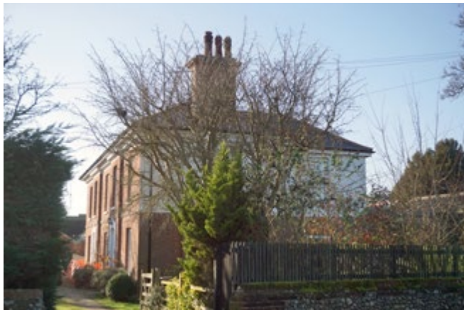
The former Police Station on Station Road
