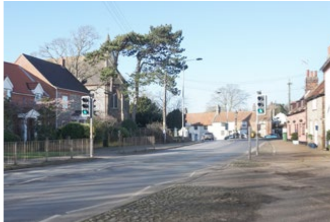
Traffic lights and basic metal railings on Norwich Road
