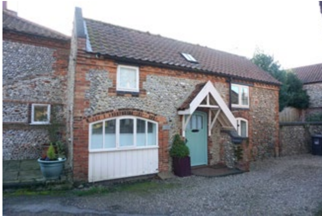
Converted outbuilding on Lees Yard
