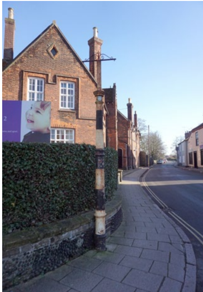
Metal signpost outside the Old School House
