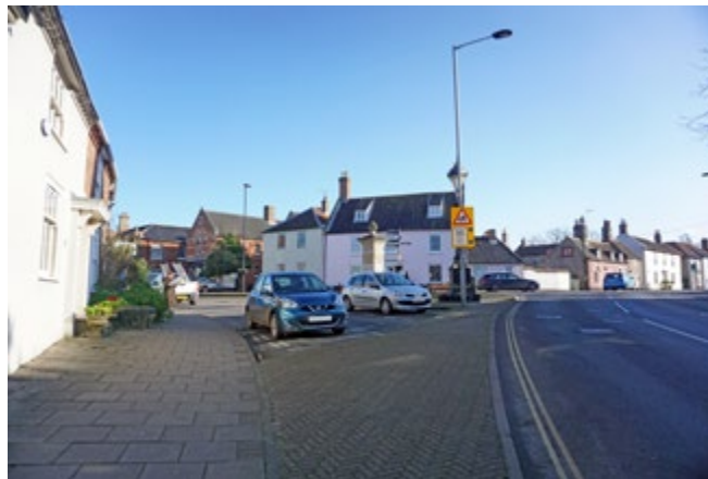
Parking and road signage at Obelisk Plain intrudes on the setting the historic obelisk and fountain/lamppost
