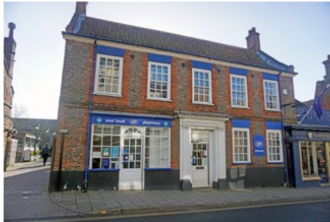
Red and brown brick to a Georgian building on the High Street, with sash windows, Classical doorcase and later inserted shop front. This building is likely to be amongst the earlier buildings to be reconstructed after the 1708 fire
