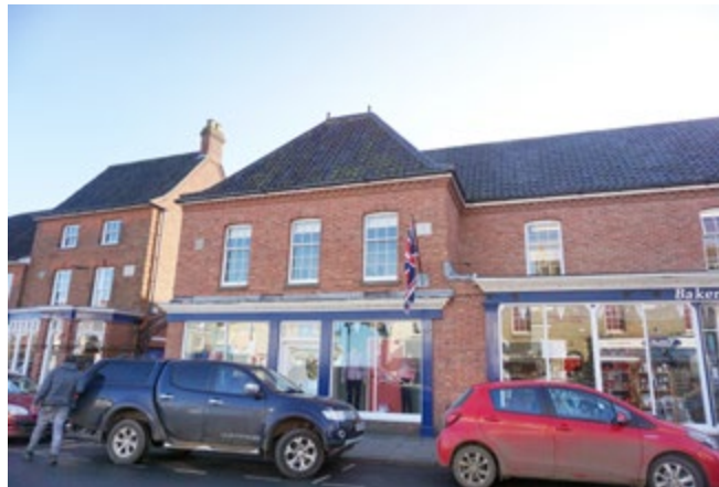
Section of Bakers and Larners on the Market Place, rebuilt in 1977
