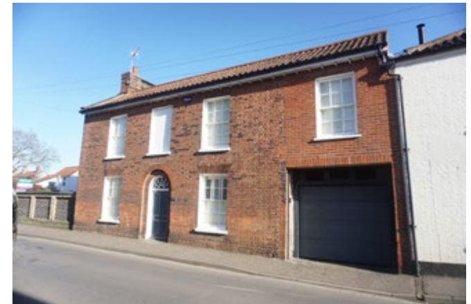
Unsympathetic garage attached to a listed building
