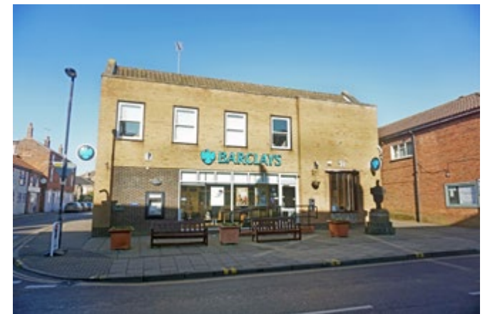
Inappropriate design of Barclays Bank on the High Street
