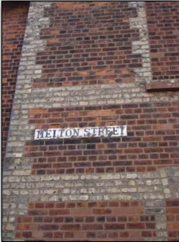
Red brick with decorative bands, Melton Street
