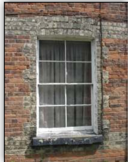
Original window detail
