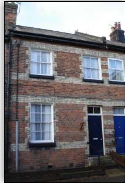
One of the few houses on Melton Street with original windows
