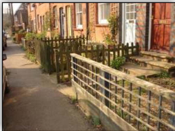
Typical enclosures to housing on Colville Road
