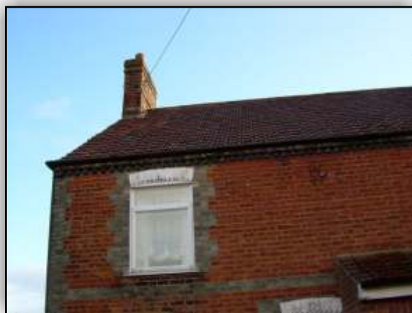
Brickwork on Kitchener Road
