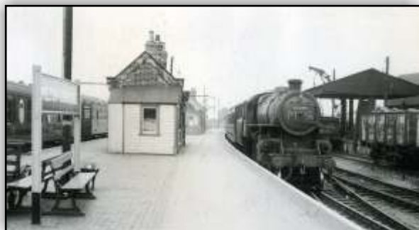
The Inspector, Foreman and Station Master's Offices on the central platform
