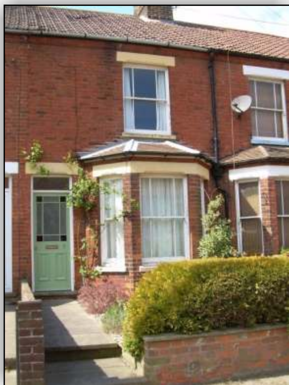
Original detailing on Kitchener Road
