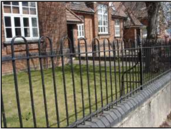
Railings outside the former school
