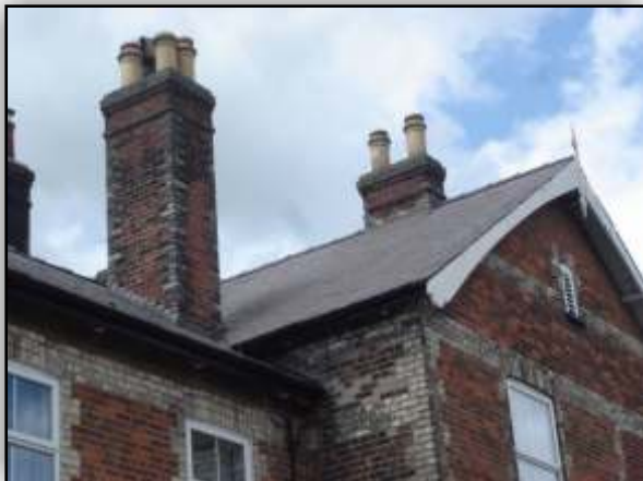
Welsh slate roofing, Melton Street
