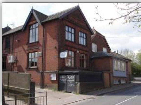
The former Railway Institute stands out on Briston Road
