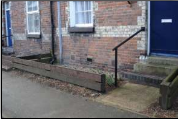
Typical threshold to dwellings on Melton Street
