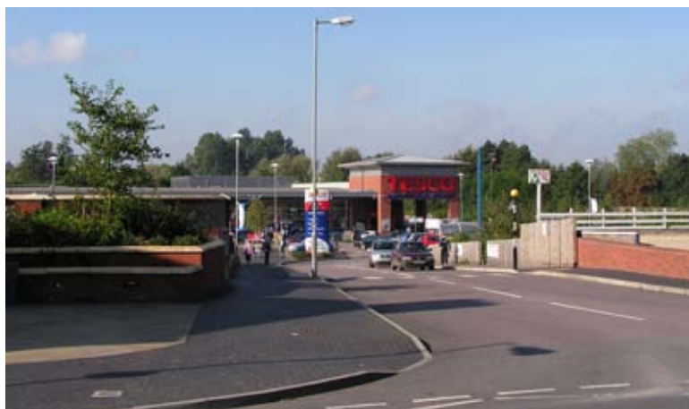
Figure 19 : Superstore entrance on Oak Street
