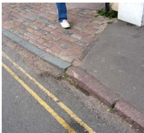
Figure 48 : Old (lower) and new granite kerbs in Bridge Street
