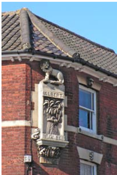
Figure 44 : Carved stonework on Albert House at the east end of Norwich Street
