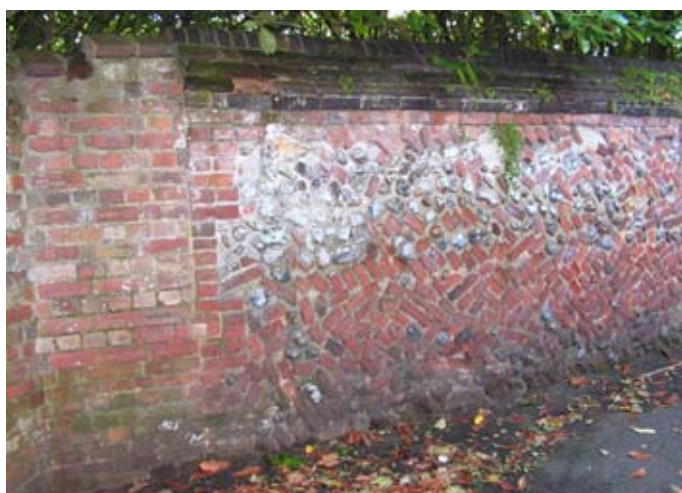
Figure 41 : Brick used as part of rubblework wall at Grove House
