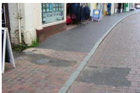
Figure 52 : Maintenance should be carried out properly. Poor replacement of surfaces in Norwich Street
