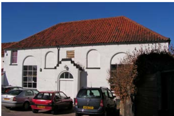
Figure 40 : Former Primitive Methodist Chapel, Oak Street
