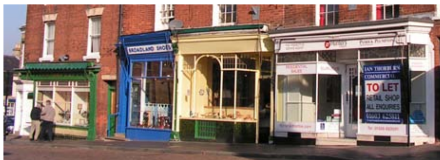
Figure 47 : Fine shop fronts on the north-west side of Upper Market
