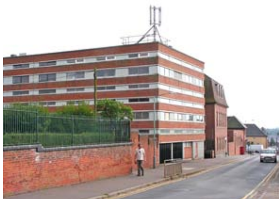
Figure 33 : Telephone exchange and Post Office depot on Queens Road
