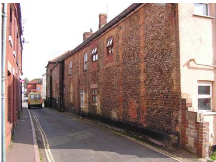
Figure 30 : Brick and flint buildings on the south side of Swan Street
