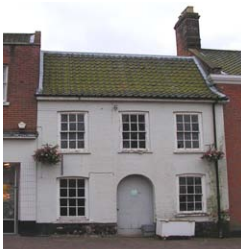
Figure 51 : Poorly maintained house on The Square
