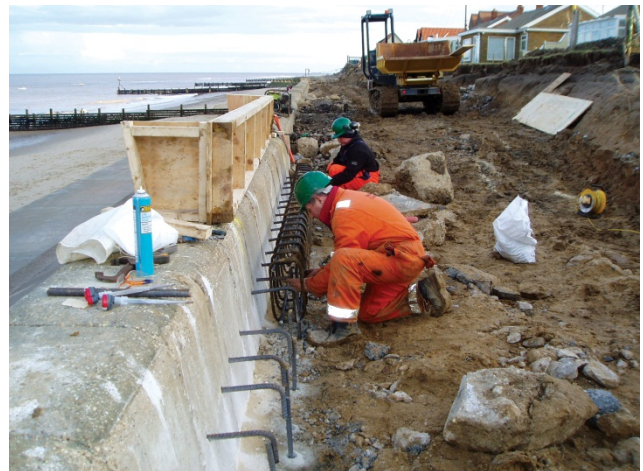
Above: Repairs taking place at Walcott
