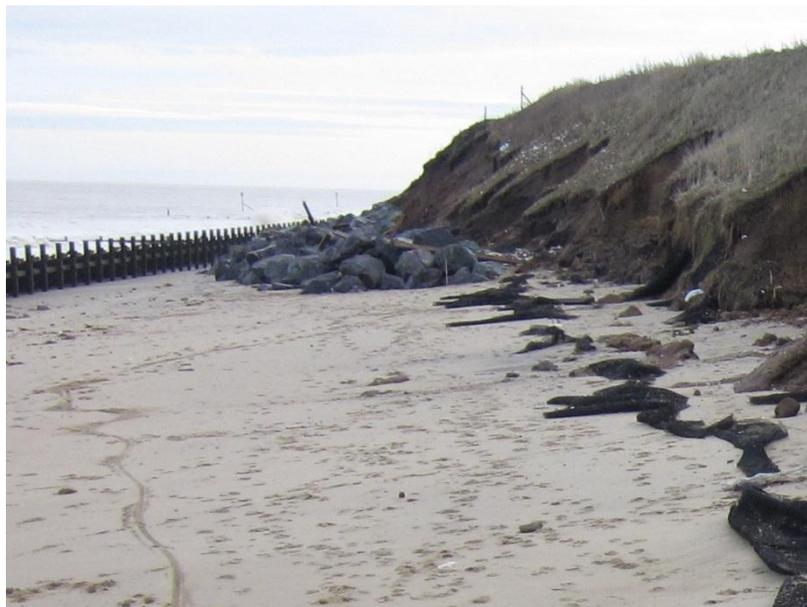
*Figure 4. Cliff erosion behind rock revetment at Bacton*
