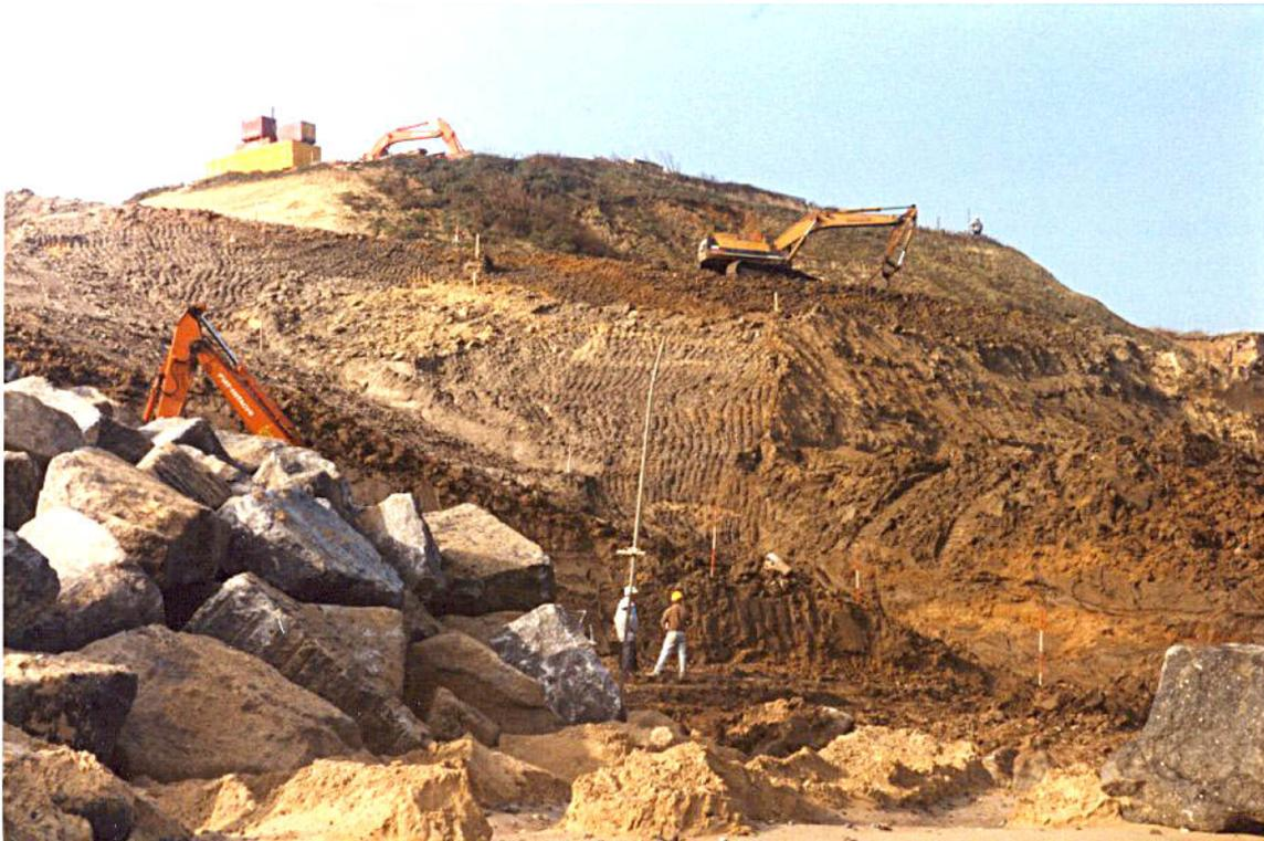
**Figure 10 - Rock Armour Toe Protection Works**
