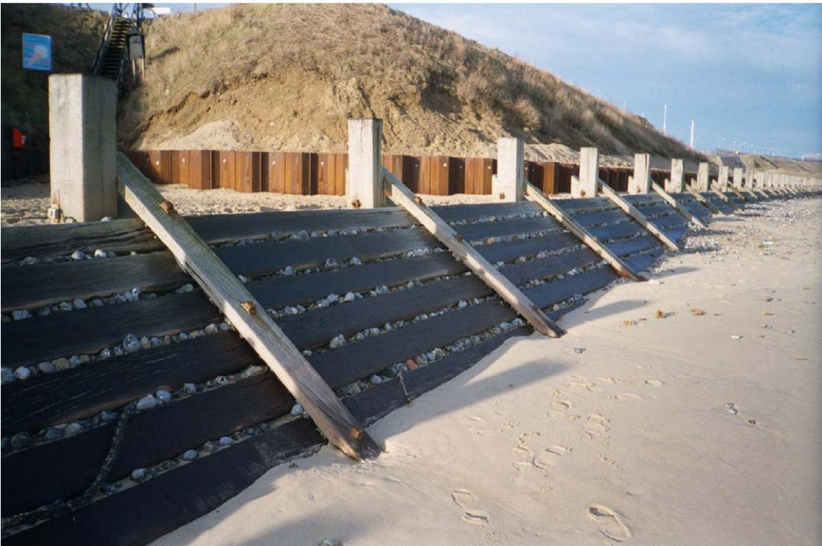
**Plate 9.5      Photo W10A      Revetment and breastwork**
