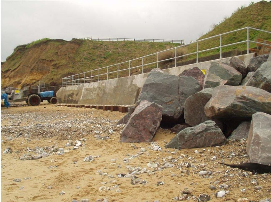
**Plate 5.11** Sea wall and rock armour outflanking revetment, west flank
