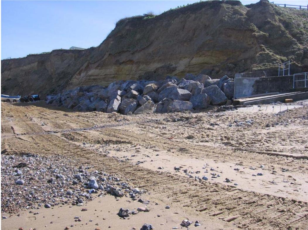
**Plate 5.9** View of rock armour revetment, east flank
