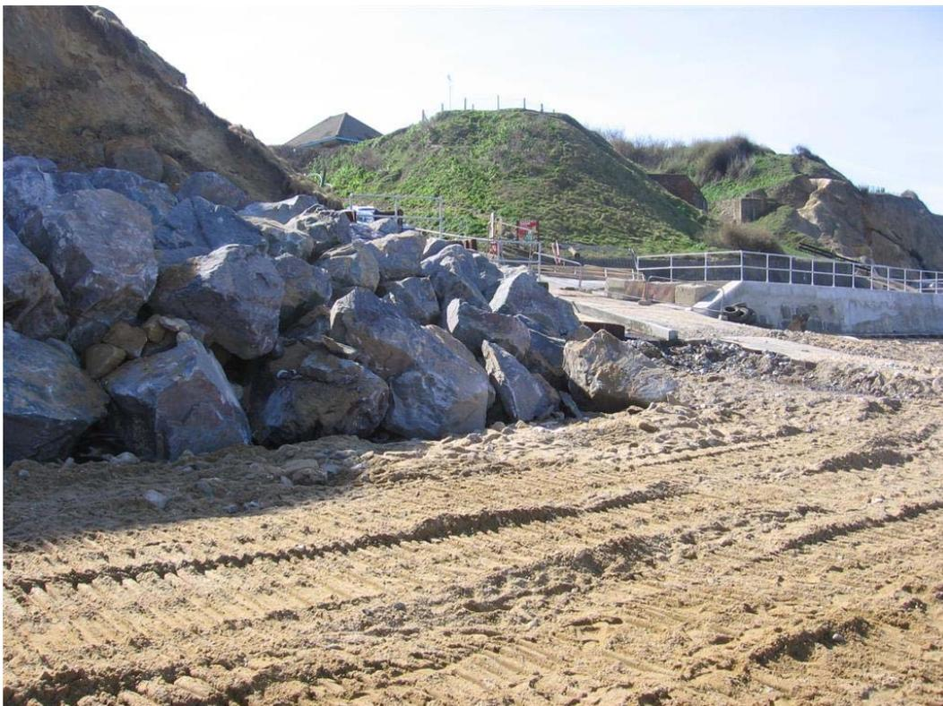
**Plate 5.10** Rock armour revetment, east flank
