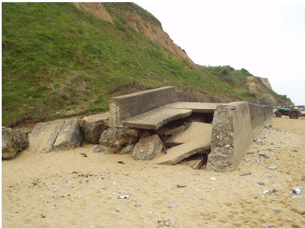
**Plate 5.7** Failure of end of west wall
