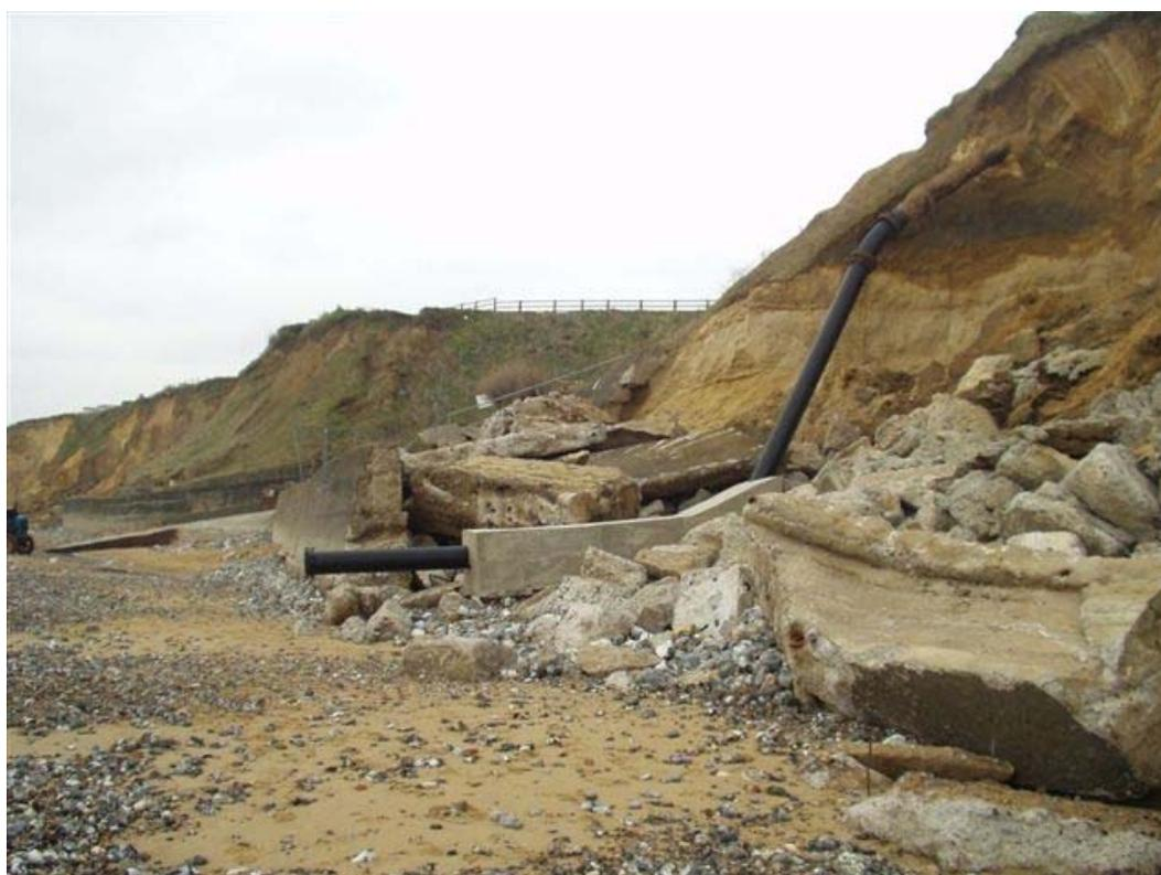
**Plate 5.8** View of the failure in east wall
