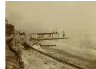
1900 – Cromer promenade/sea wall and pier under construction
