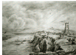
1822 – Slumping and overhanging cliffs with little protection from the sea
