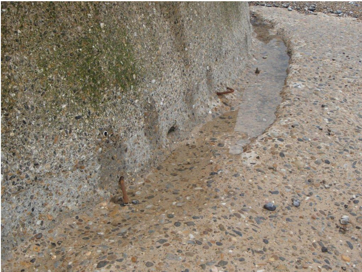
Concrete worn away by the action of the sea, 2013. NNDC Image.
