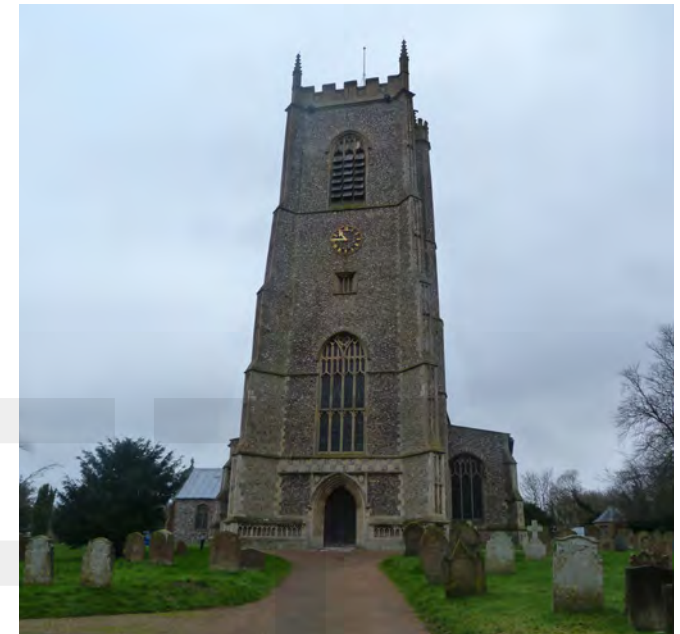
Blakeney Parish Church
