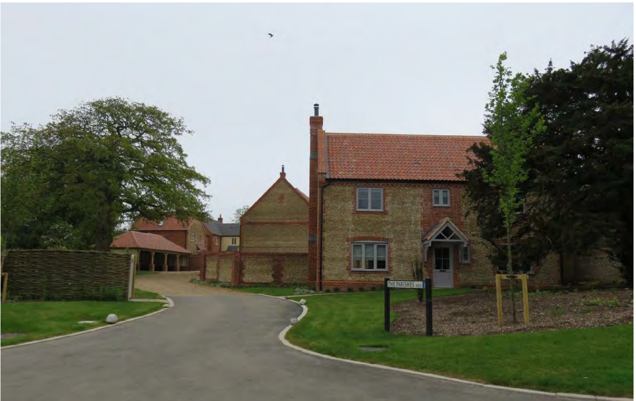
New in-fill housing at Weybourne.
