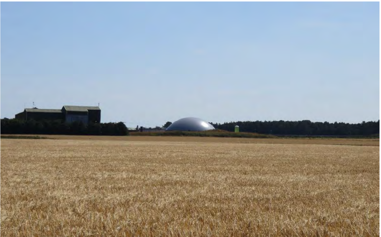
The anaerobic digestion plant at Egmere.
