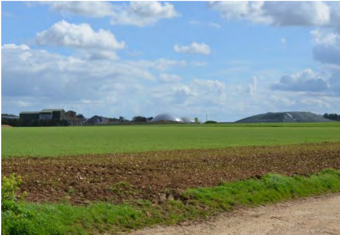
Figure 3.8: Existing AD plant at Egmere, with feedstock storage mound in right of image.
