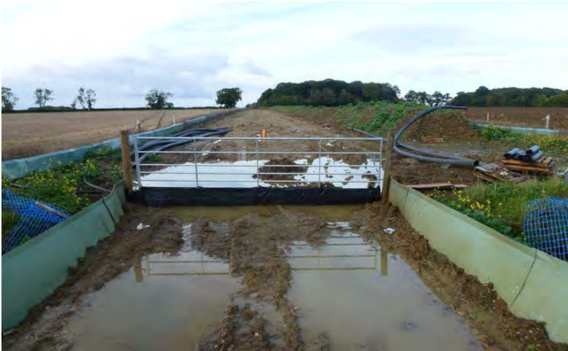
Figure 3.5: Cable trench for the Dudgeon offshore wind farm near Stanfield, Norfolk
