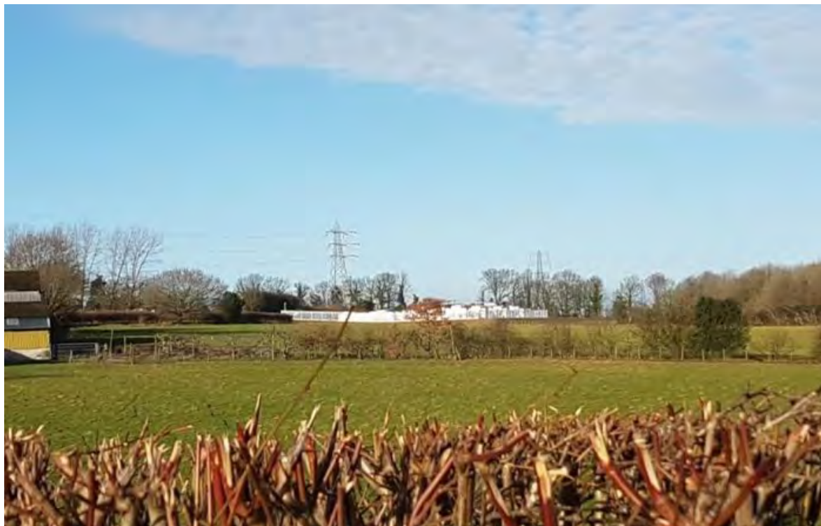
Figure 3.7: A view of the recently constructed Glassenbury battery storage compound in Kent (centre, background of image), which occupies a site area of 0.9 ha and features buildings/equipment up to 5m in height
