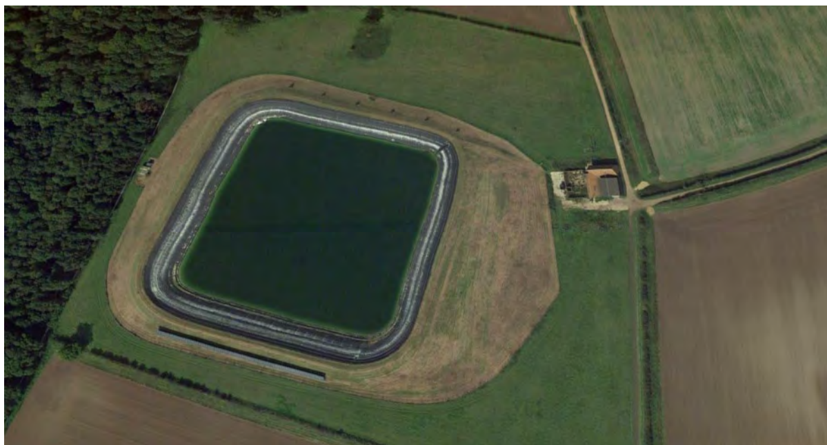
Figure 3.9: Reservoir at Holkham (total area approx 5 ha), showing grassed embankments and rubber lining.
