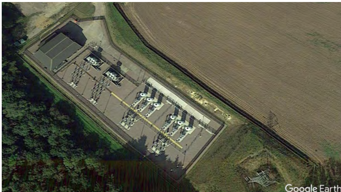
Figure 3.6: Substation for the Sheringham Shoal offshore windfarm near Salle, Broadland District
