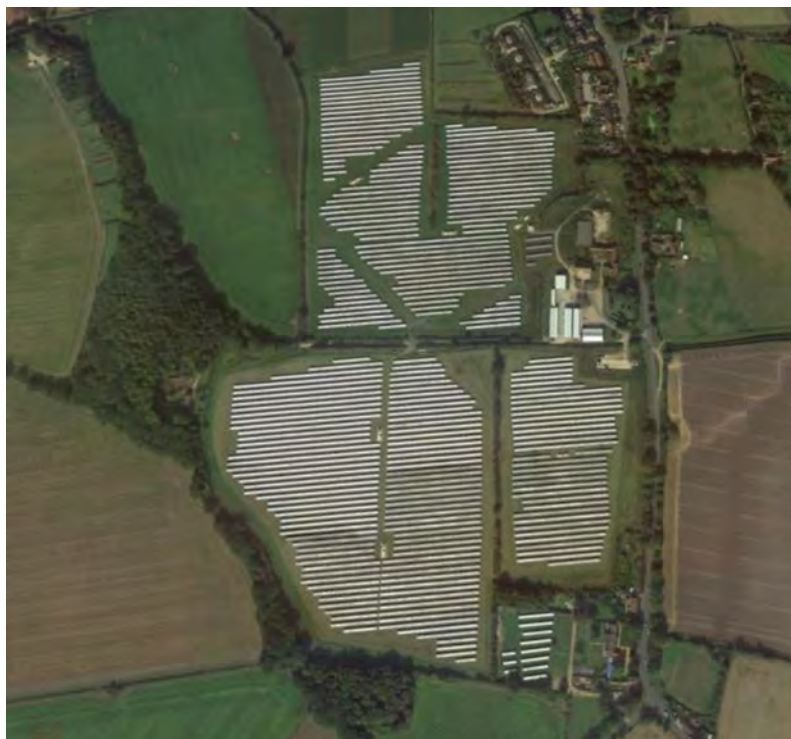
Figure 3.4: A 10MW solar PV development occupying a 27 ha site in Northrepps, North Norfolk
