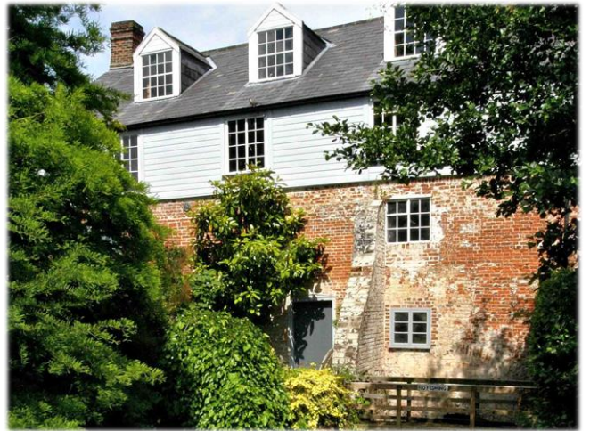
8. The Mill showing wooden cladding, brick with classical dormer windows
