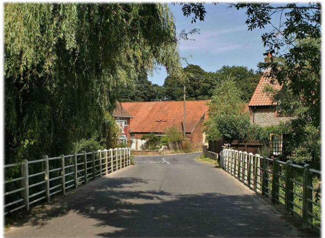
20. Bridge railings over the Bure between Saxthorpe and Corpusty
