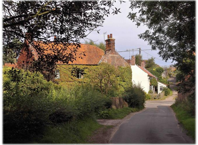
14. Eclectic architectural view showing gable-ends, chimneys lean-to extension and surrounding greenery
