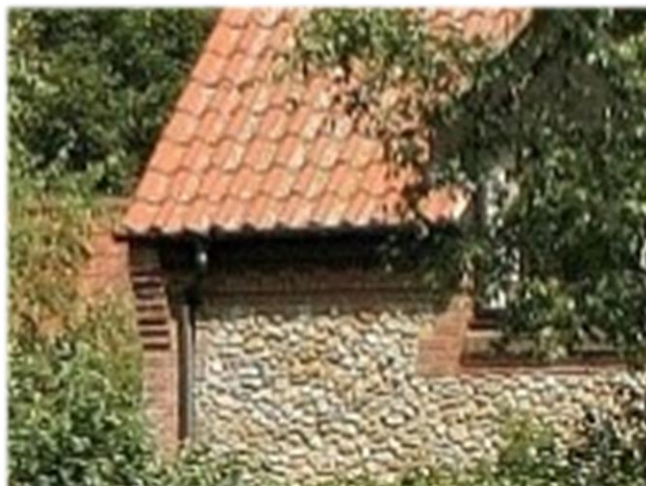
2. Brick and flint construction with pantile roof
