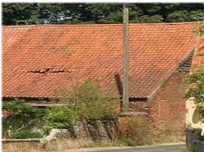
1. Brick with pantile roof
