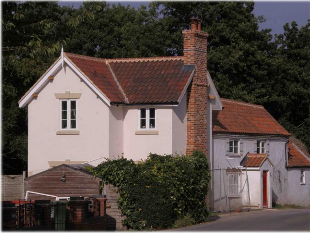
17. Modern extension to cottage retaining original features and sympathetic use of stucco
