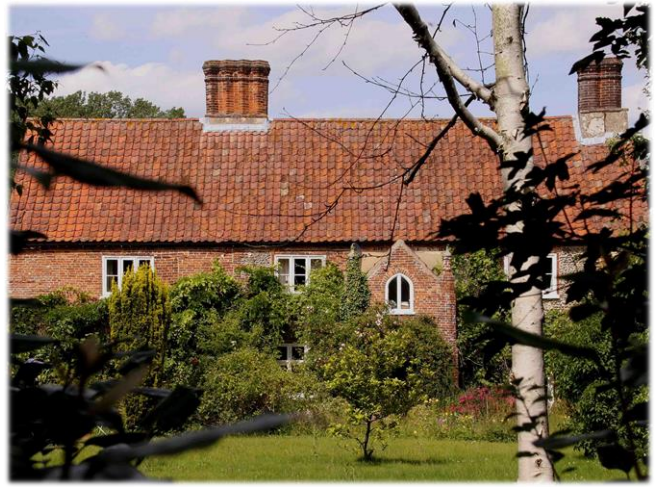
10. 16 th Century brick and pantile Manor House, Corpusty
