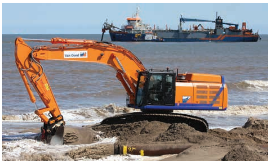
A dredger and excavator similar to those which will be used during the Sandscaping scheme.
