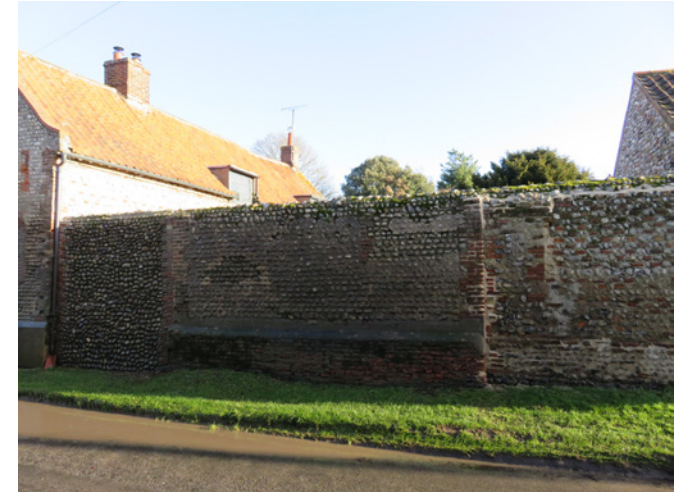
Grade II listed wall to Green Farm
