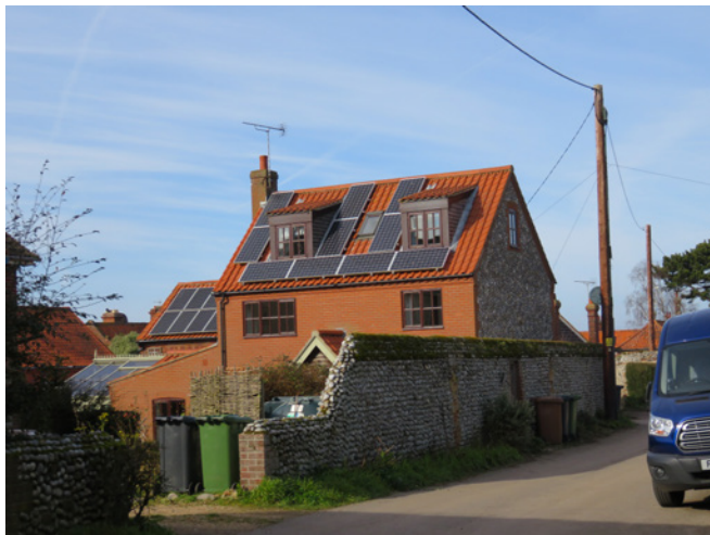
Prominent solar panels detract from the character of the conservation area
