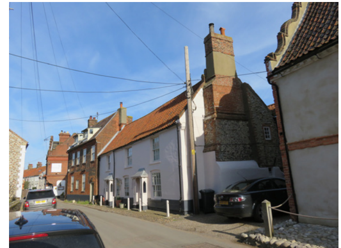
Profusion of electricity and telegraph cables across the High Street
