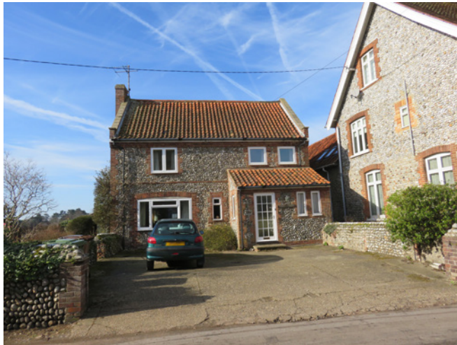
Front garden replaced with concrete. Not only does the concrete surface detract from the Conservation Area but also the loss of a boundary demarcation.
