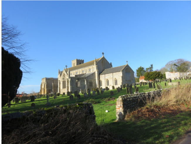
View from the southern gate to the churchyard from Church Lane looking towards the church
