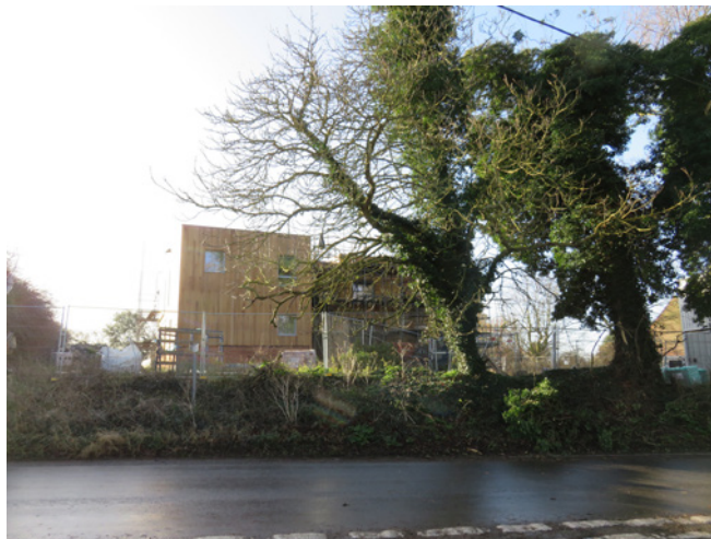
The scale and massing of this new dwelling are out of keeping with the other dwellings around Cley Green and significantly detracts from views around the Green as well as the setting of the church and nearby historic buildings
