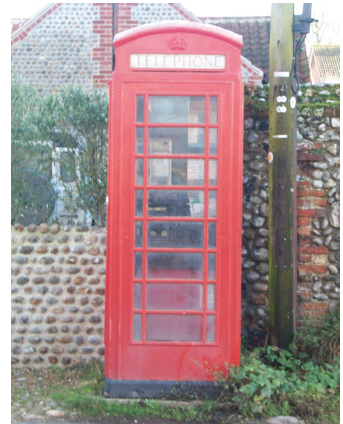
K6 Telephone box, Grade II Listed
