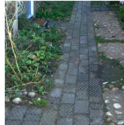
Detail of the paving to the footpaths
