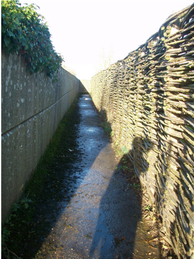
Concrete walling to footpath at west of High Street
