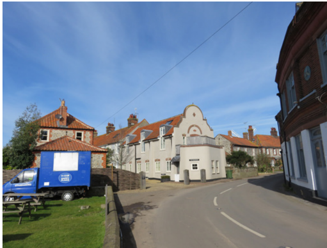
View south down the High Street
