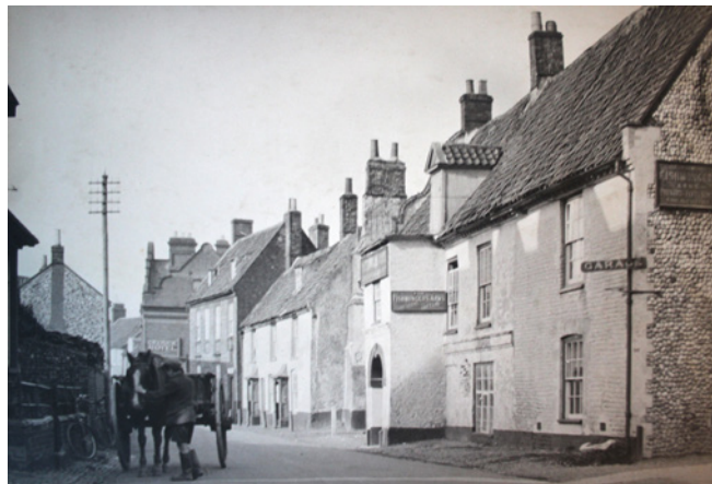
View of the High Street with the Fishmonger's Arms and the George Hotel, 1931 (Image courtesy of Norfolk Heritage Centre, Norfolk and Norwich Millennium Library: C/CLE 5525)
