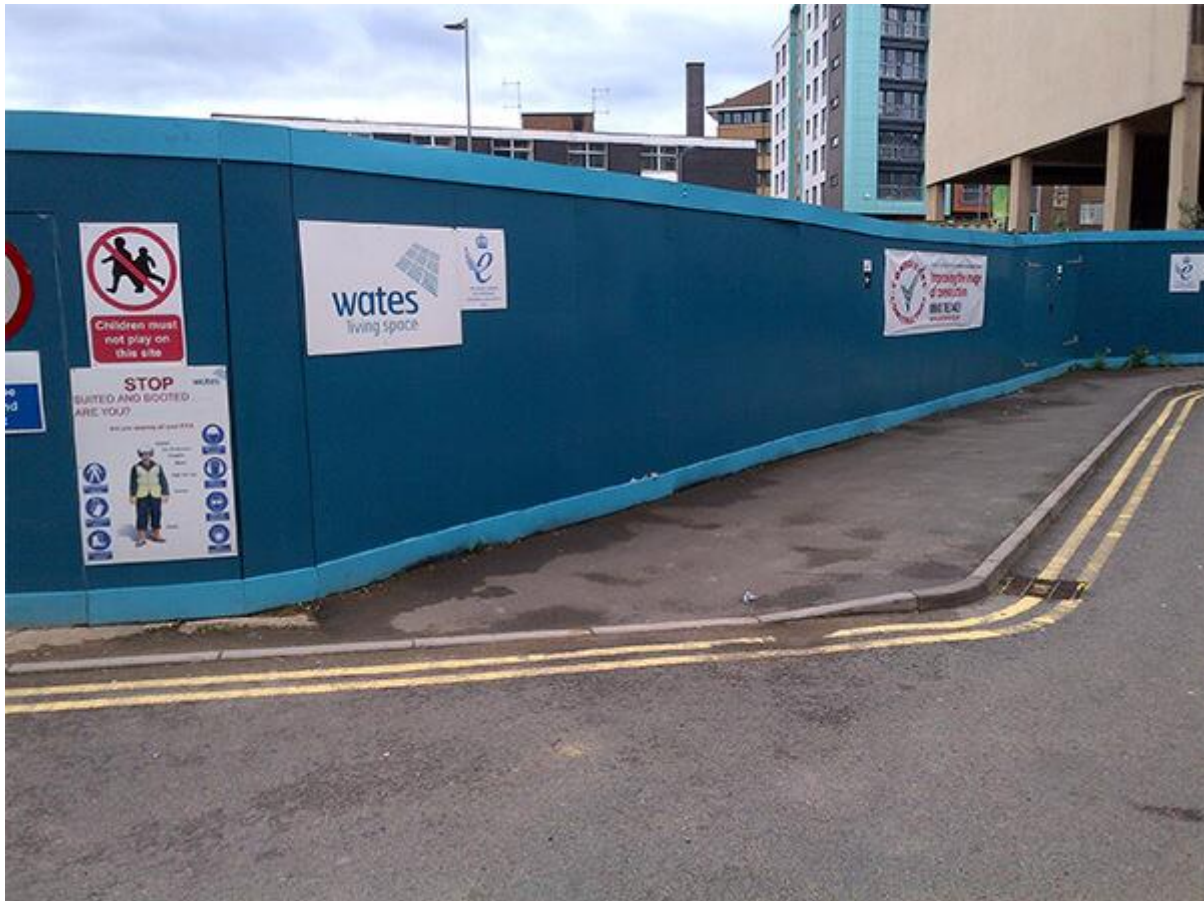
Photo 1. Example of solid hoarding
