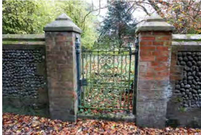
Decorative metal pedestrian gates in a brick and flint wall to Hempstead Lodge
