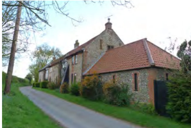
Old Church Barn/The Great Barn
