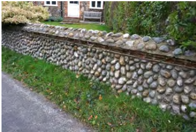
Flint cobble wall
