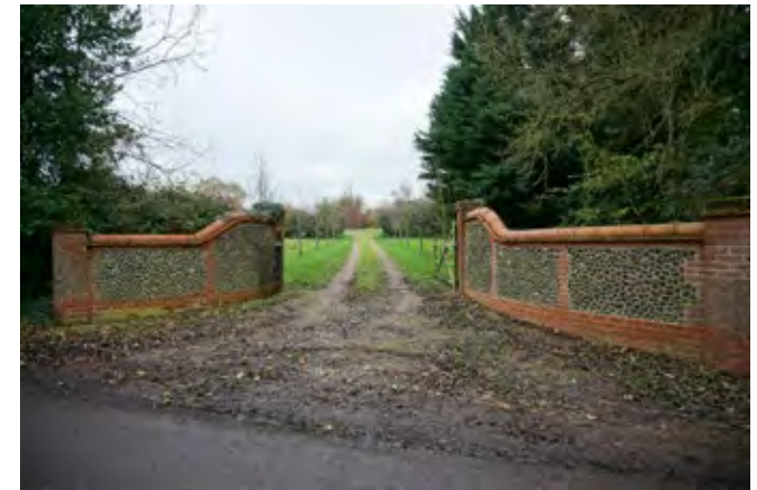
Flint and brick flank walls to a gate
