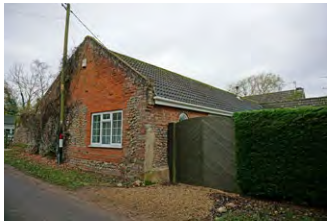
Converted agricultural building at Church Farm
