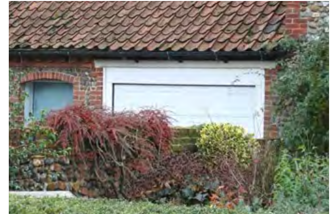
Modern garage doors inserted into historic fabric
