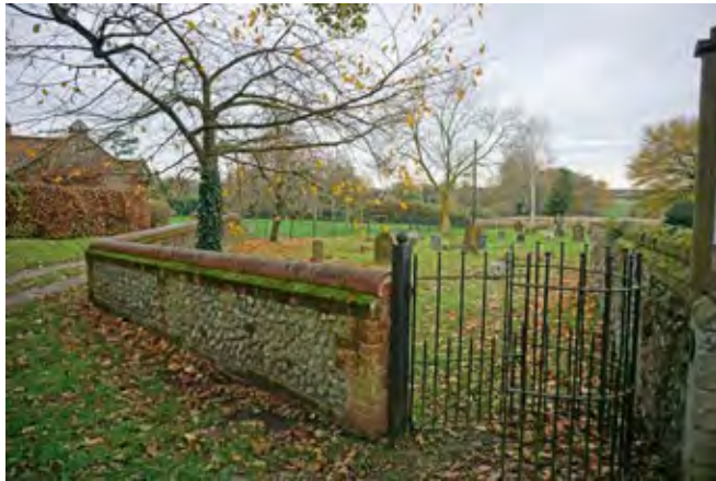
Wall, fences and kissing gate to the graveyard
