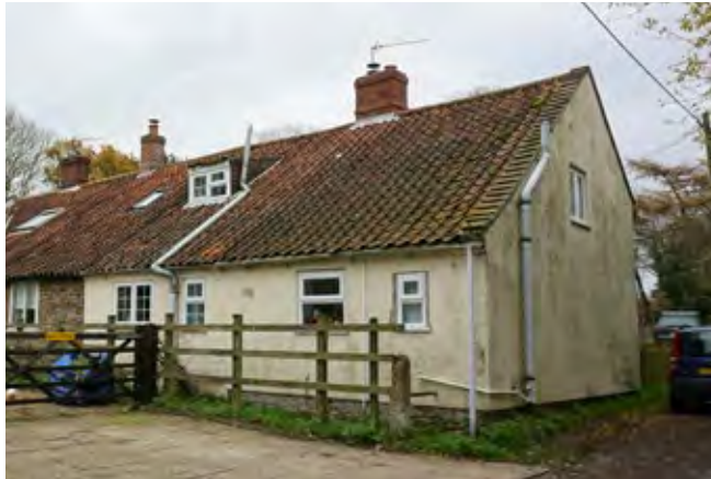
Inappropriate and cluttered uPVC downpipes/ventilation pipes in a light colour
