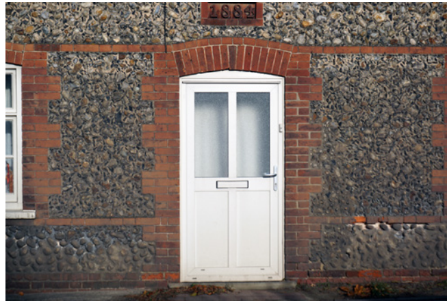
Inappropriate uPVC door
