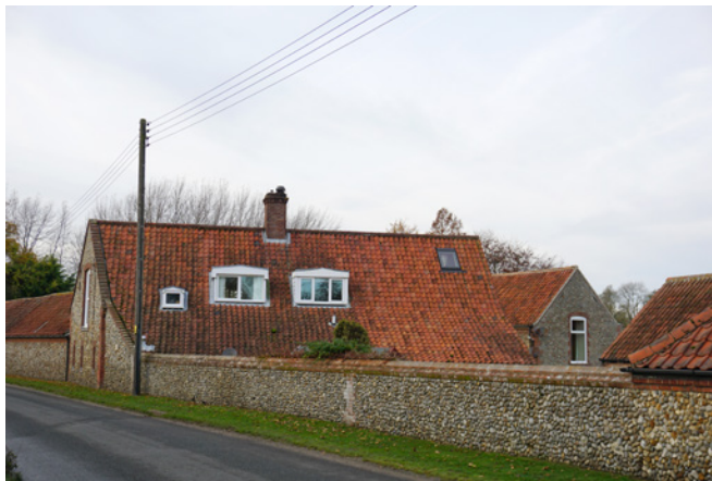
Converted barn at Home Farm
