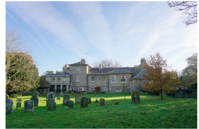
West elevation of Letheringsett Hall, seen from the churchyard
