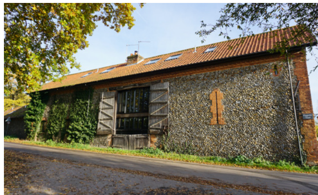
Converted Pigotts Barn on Riverside Road
