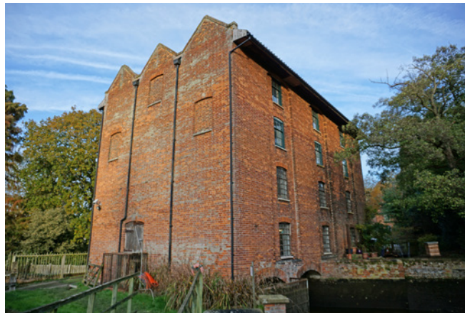
Letheringsett Mill, west and south elevations
