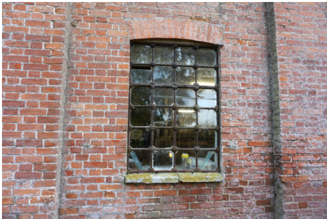
Rusting and bowed window on the mill
