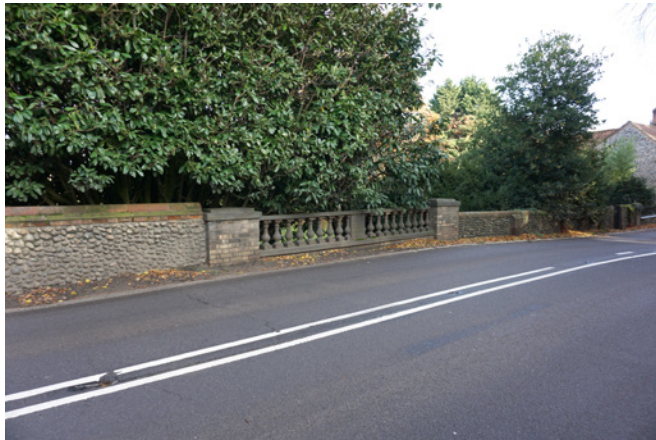
Flint and brick walls with carved stone columns to the bridge on Holt Road
