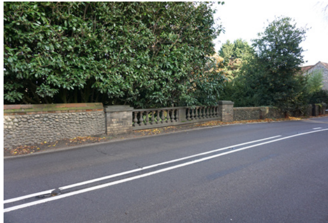
Dirty stonework to the bridge on Holt Road, also showing the lack of pavement at this point on the road
