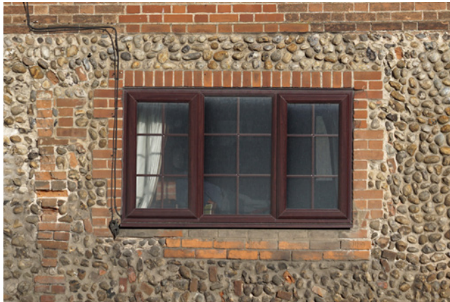
Inappropriate uPVC window
