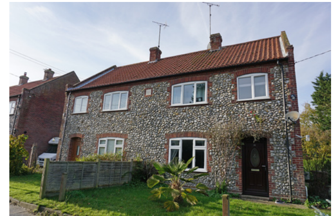
Modern cottages on Riverside Road
