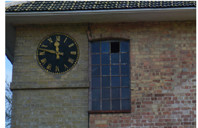
Rusting window frame with glass pane missing
