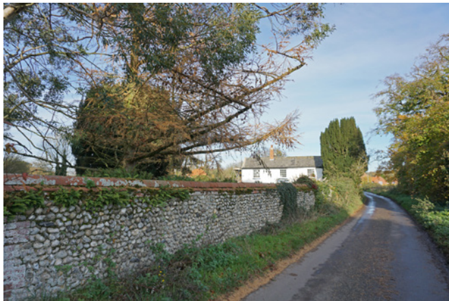
Flint and brick wall on Riverside Road
