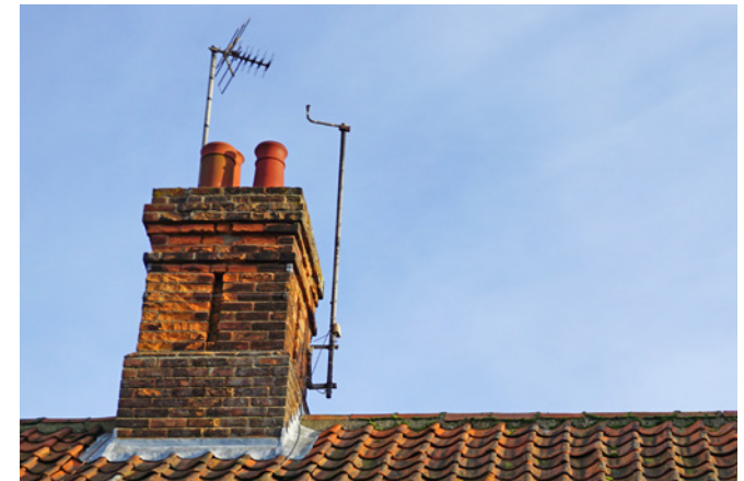
Eroding brickwork on a chimney
