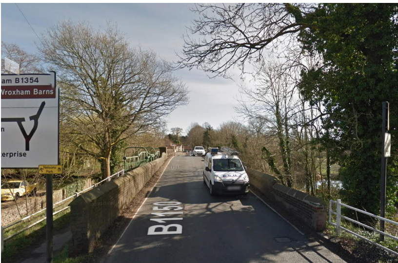
Figure 2 – B1150 Coltishall Bridge
