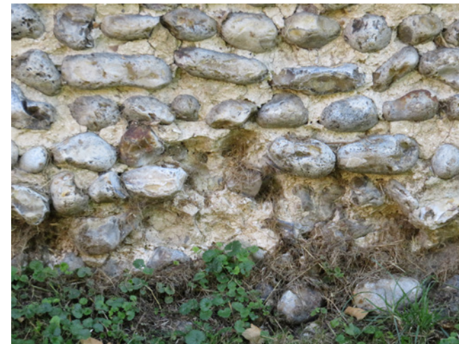
Eroded pointing causes loss of flints
