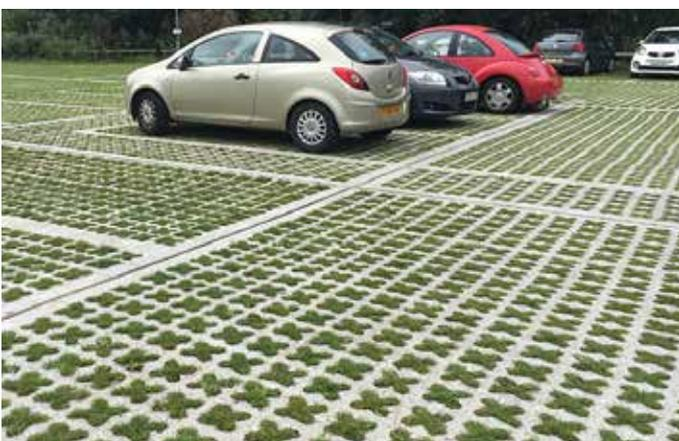
Figure 28: Examples of permeable sustainable materials that are durable and can manage surface water run-off. (Source: <https://gridforce.co.uk/car-parks>).
