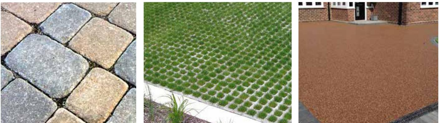
Figure 98: Examples of permeable paving that can be used in the front and rear gardens of residential buildings.
