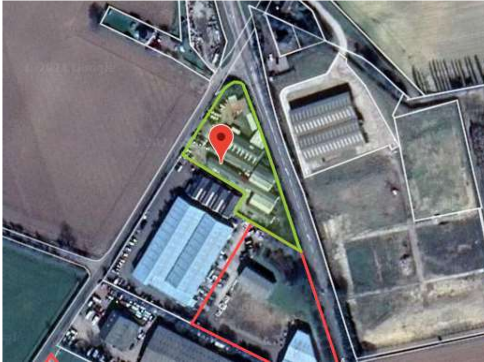
Figure 21 – Entry-point Landholding at Catfield Industrial Estate
