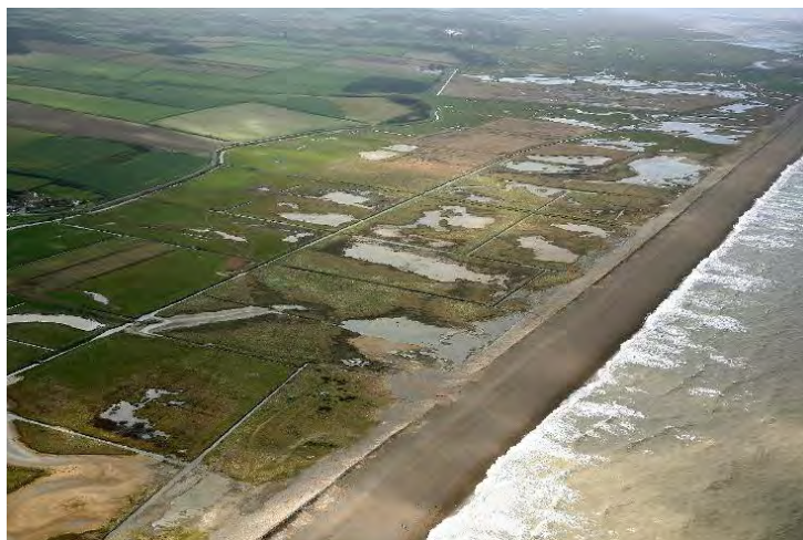
Photo 2.12: Overtopping at Salthouse (April 2007)
