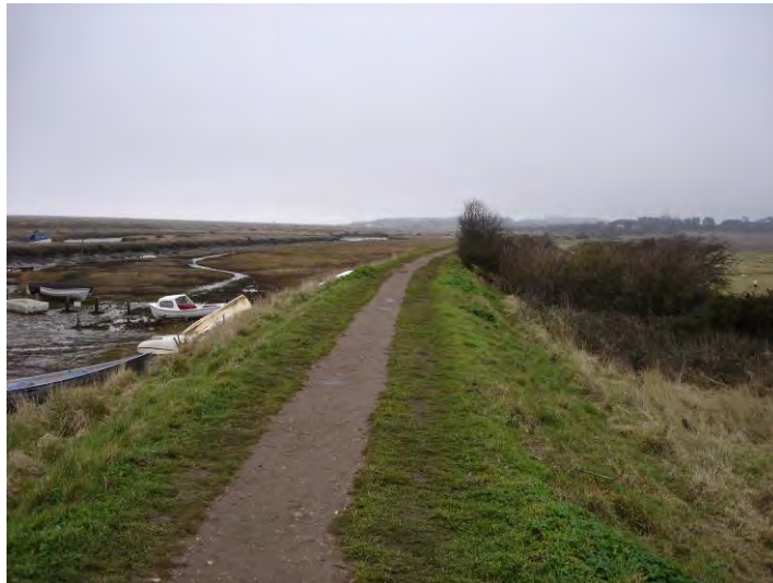
Photo 2.6: Morston flood embankment
