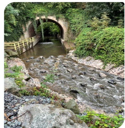
Kingfisher bridge, with fish barrier removed
