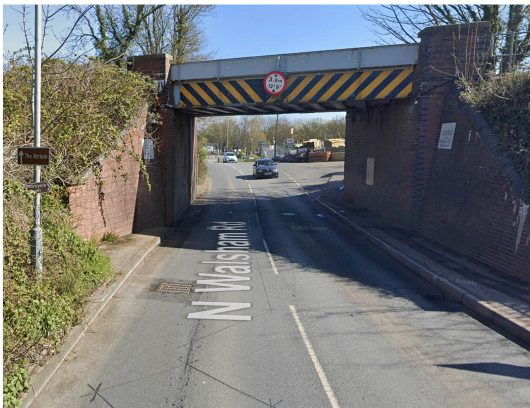
Figure 5-2 – Height restriction on N Walsham Rd
