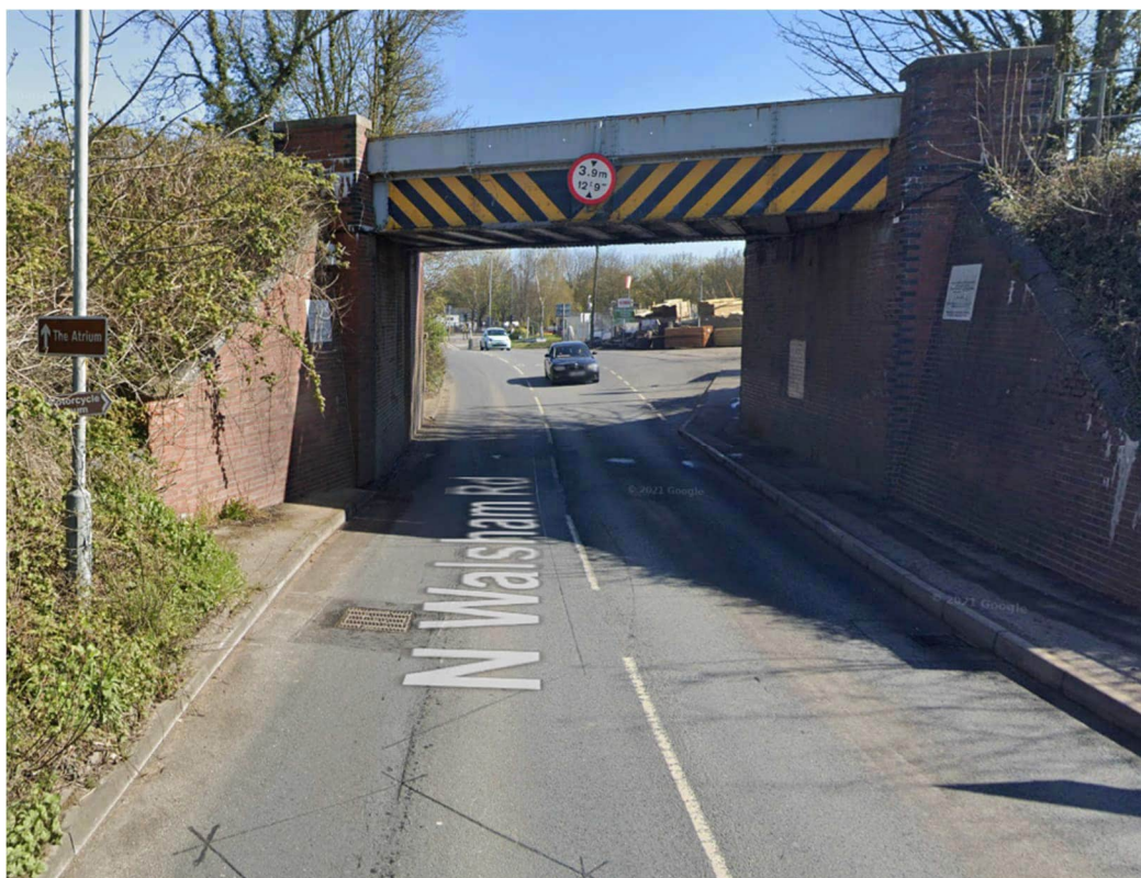
Figure 5-2 – Height restriction on N Walsham Rd
