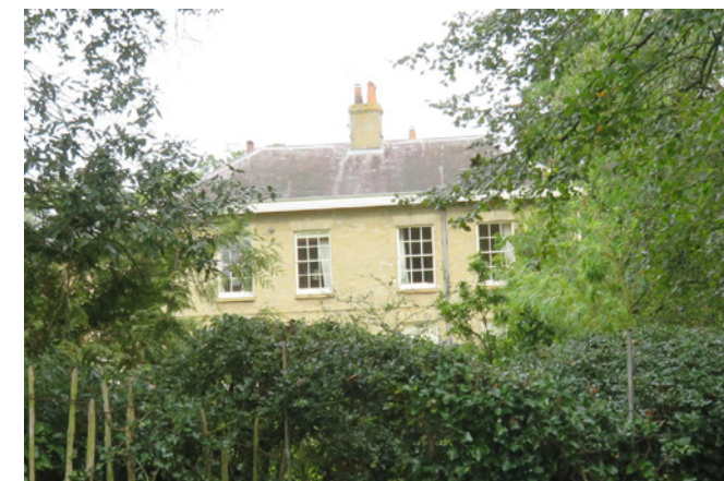
The remodelled Brinton Hall
