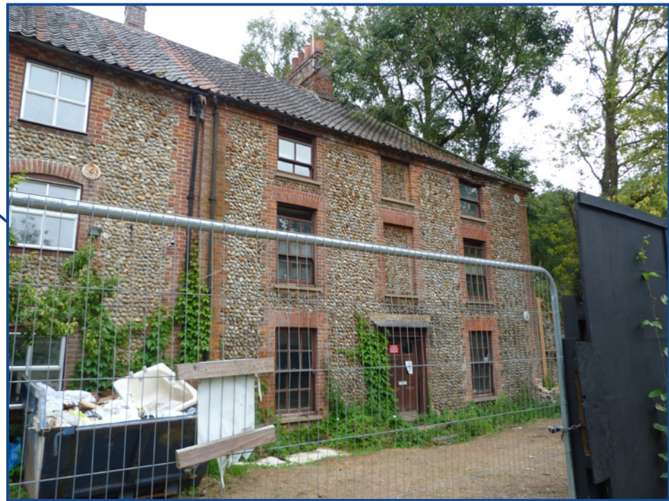
Hempstead Mill (also known as Holt Mill)
