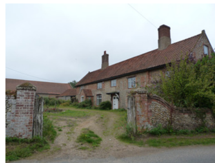
Farmhouse at Green Farm near Hempstead
