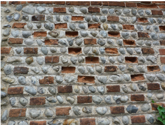
Cobbled flint and red brick patterning, with cement mortar
