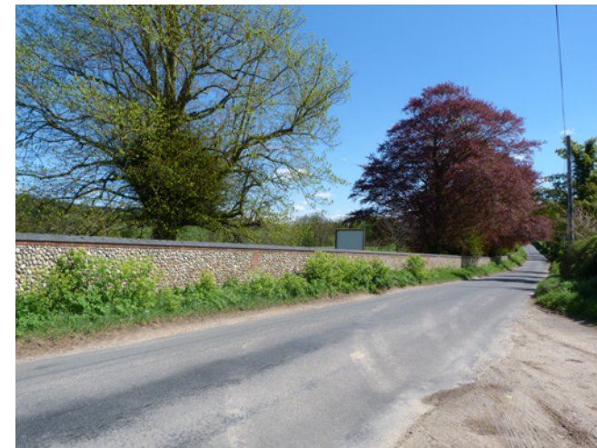
Wall bounding the Bayfield Hall site
