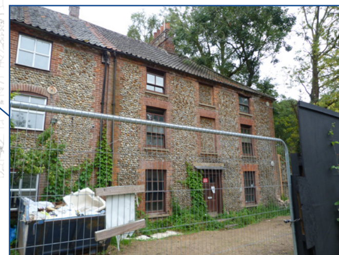
Hempstead Mill (also known as Holt Mill)
