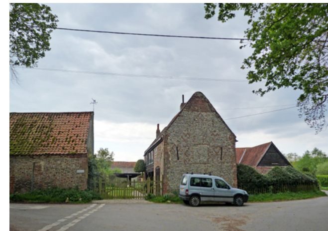
Converted agricultural buildings in Hunworth
