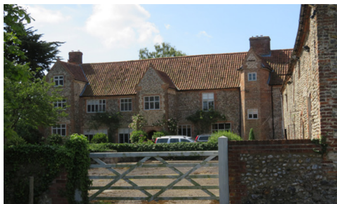
Front elevation of Sharrington Hall
