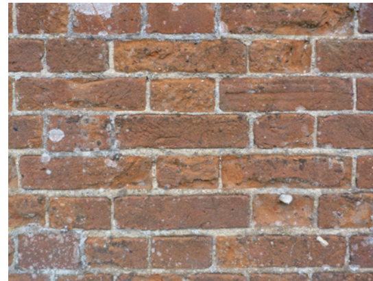
Red brick with lime mortar
