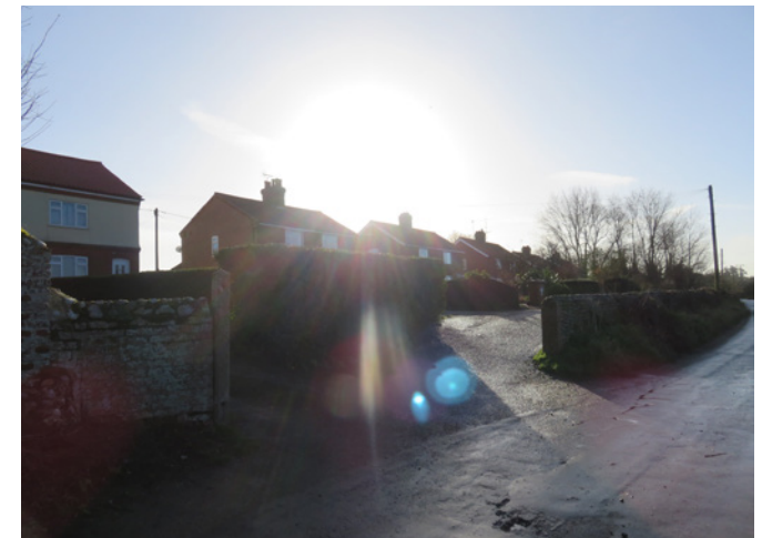
Mid-twentieth century semi-detached houses south of Cley
