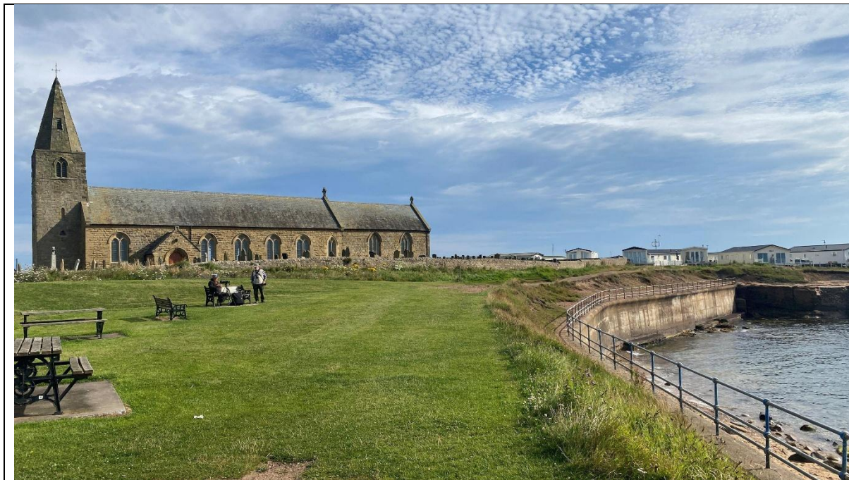
Figure 3-3: St Bartholomews Church, Newbiggin. Source: BBC (2024) 7
